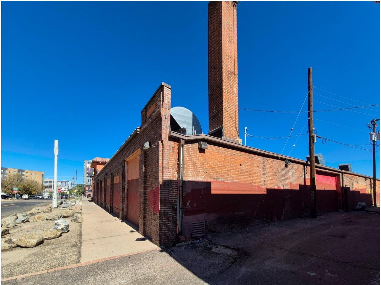
Image 4: California Street Garage, southeast elevation (2025)
