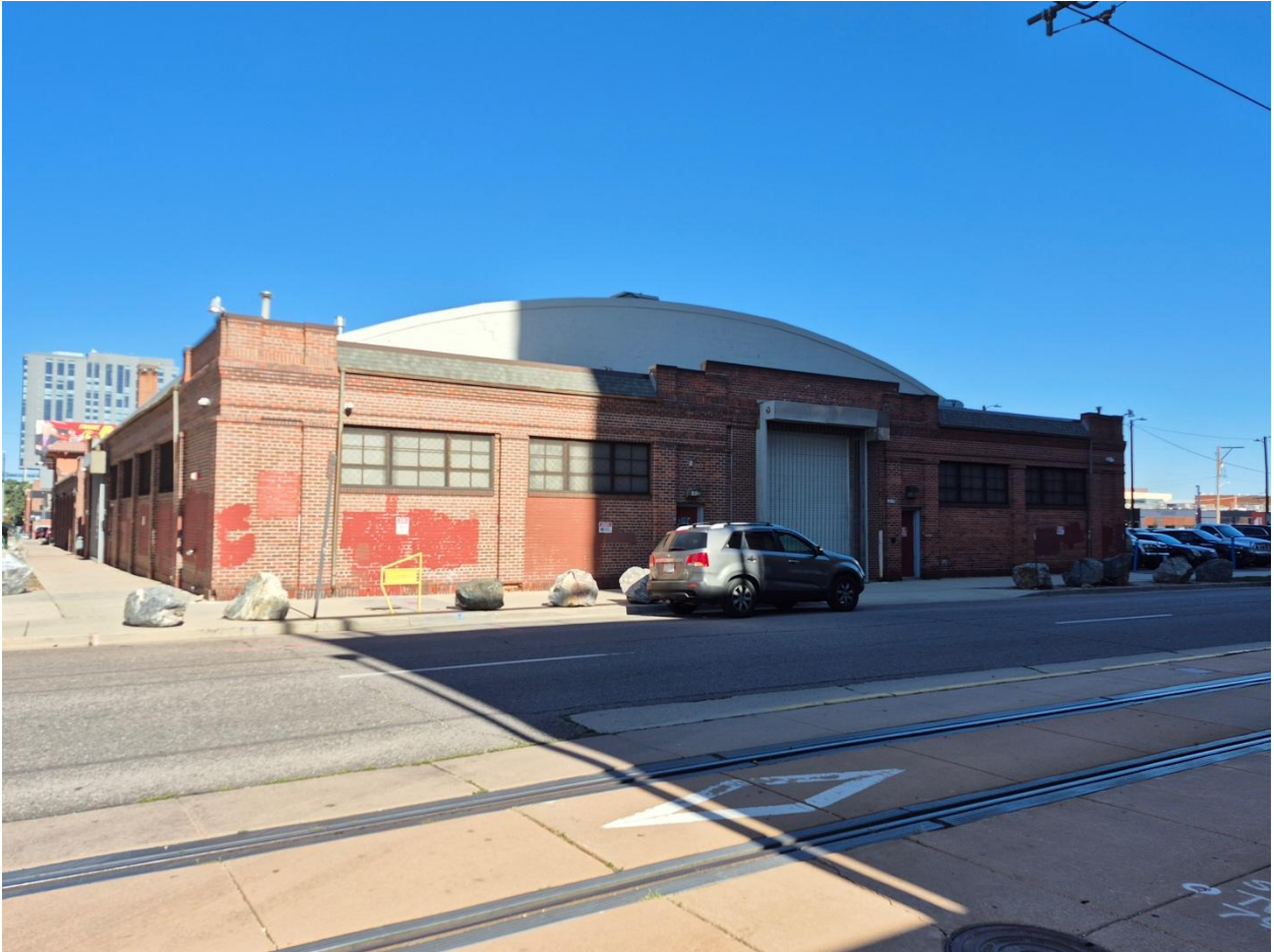
Image 6: Welton Street Garage, southeast elevation (2025)
