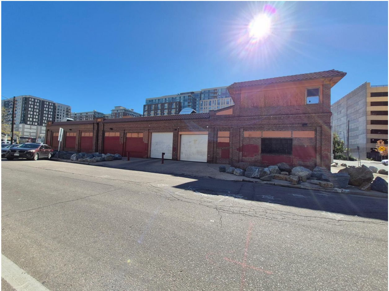
Image 2: California Street Garage, northwest elevation (2025)
