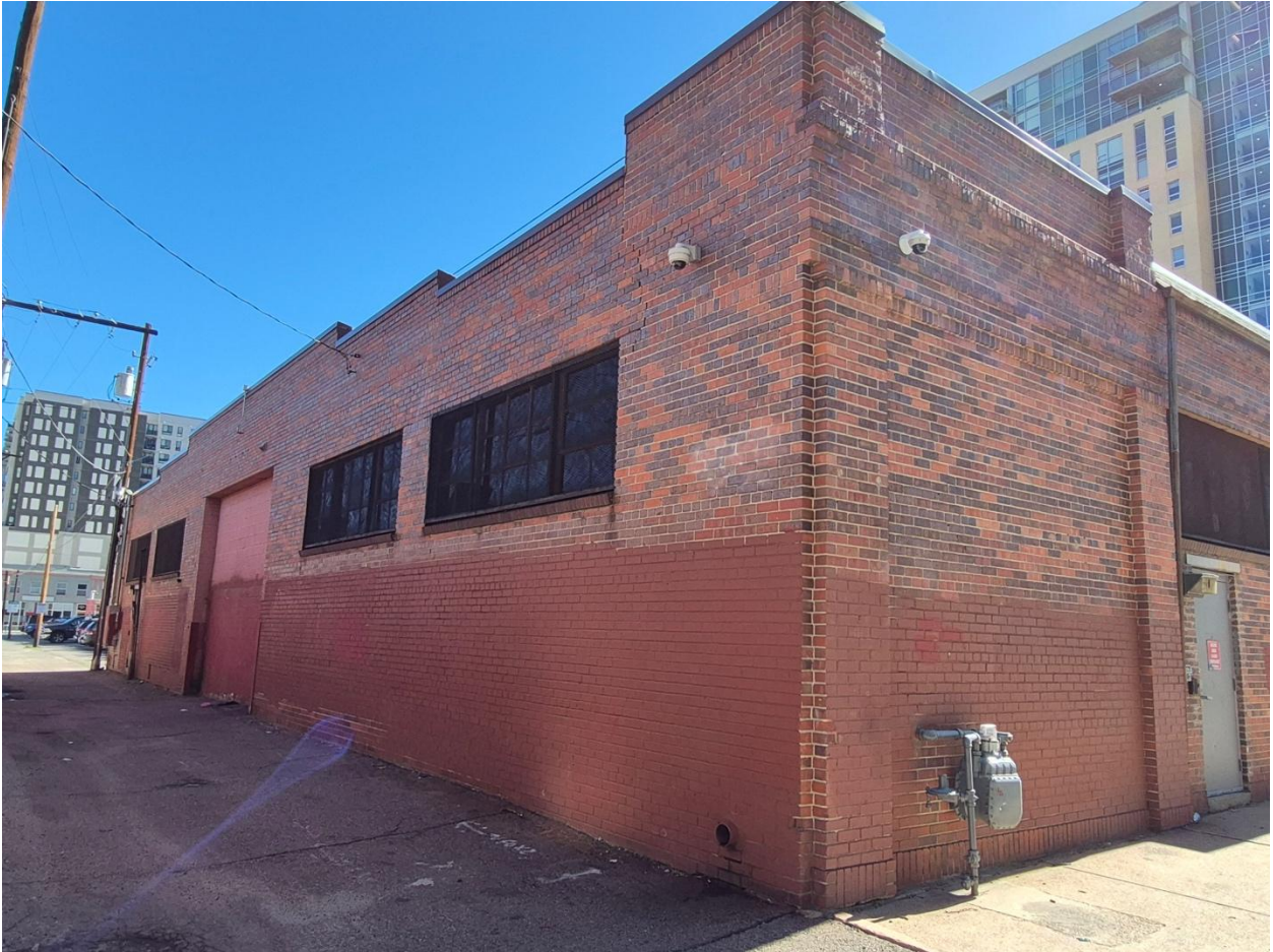
Image 7: Welton Street Garage, northwest elevation (2025)
