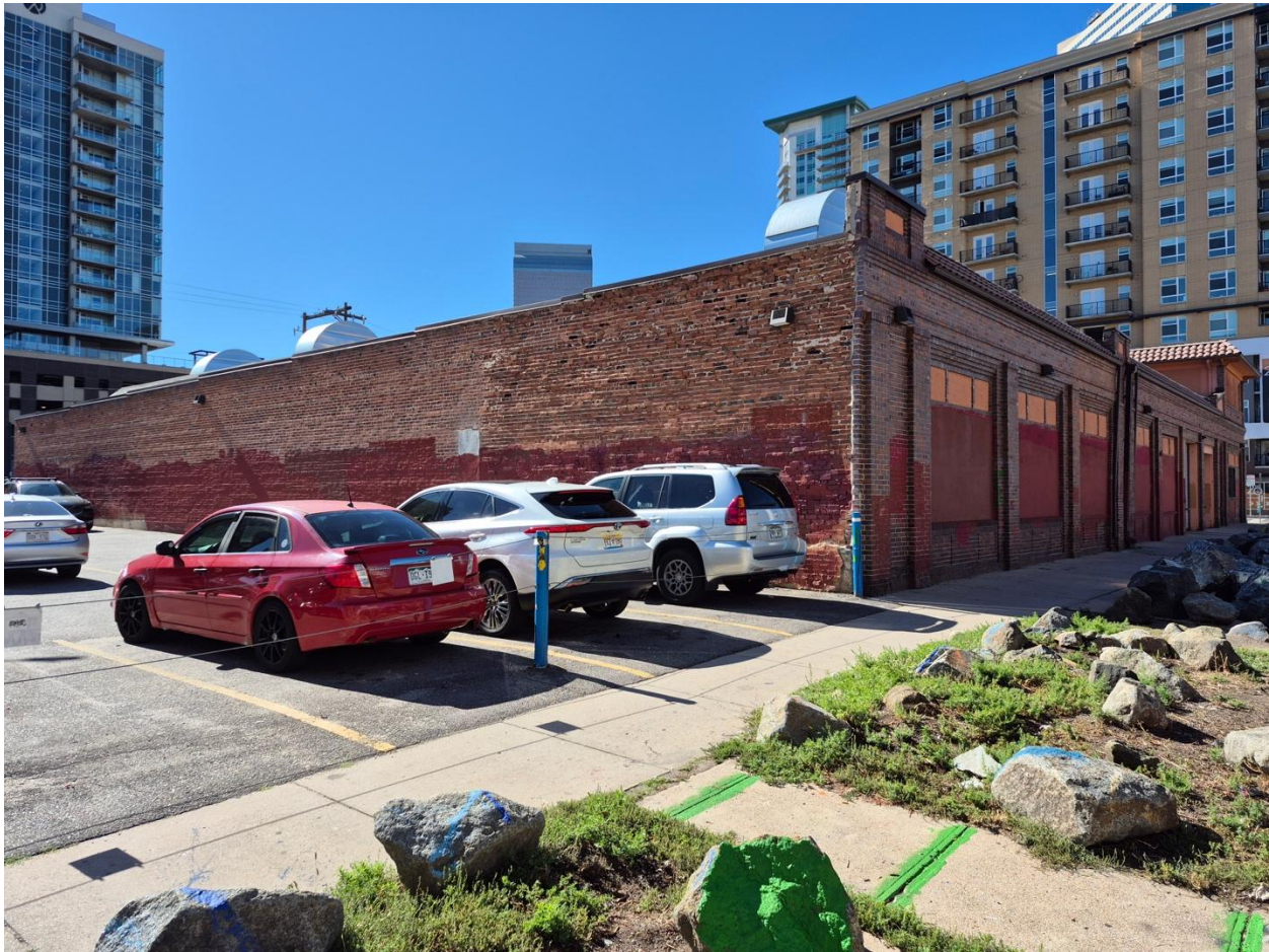
Image 3: California Street Garage, northeast elevation (2025)
