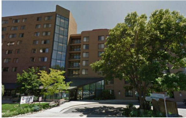
Subject site looking directly east to the front entrance and link between the older nine-story building at 22 South Adams Street and newer seven-story building at 44 South Adams Street.
