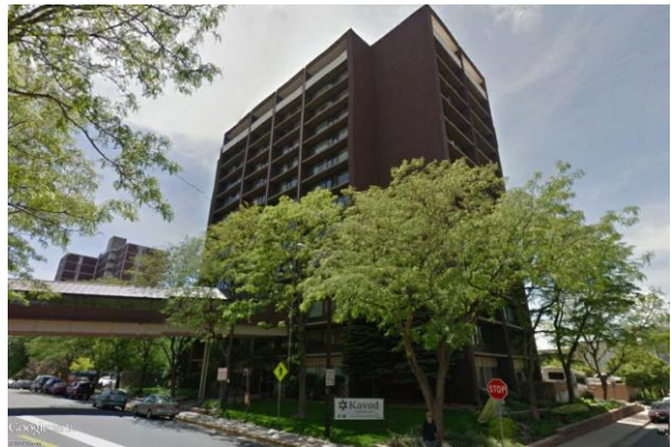
15-story building at 11 South Adams that is connected to the subject site (not visible at left) by a second-story pedestrian bridge.
