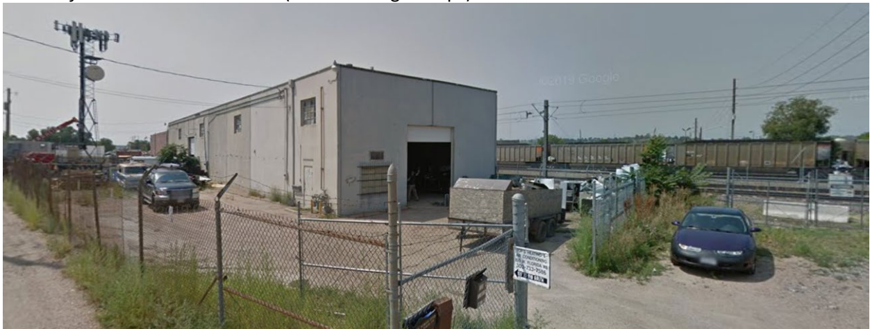
West – from West Florida Avenue (Source: Google Maps)
