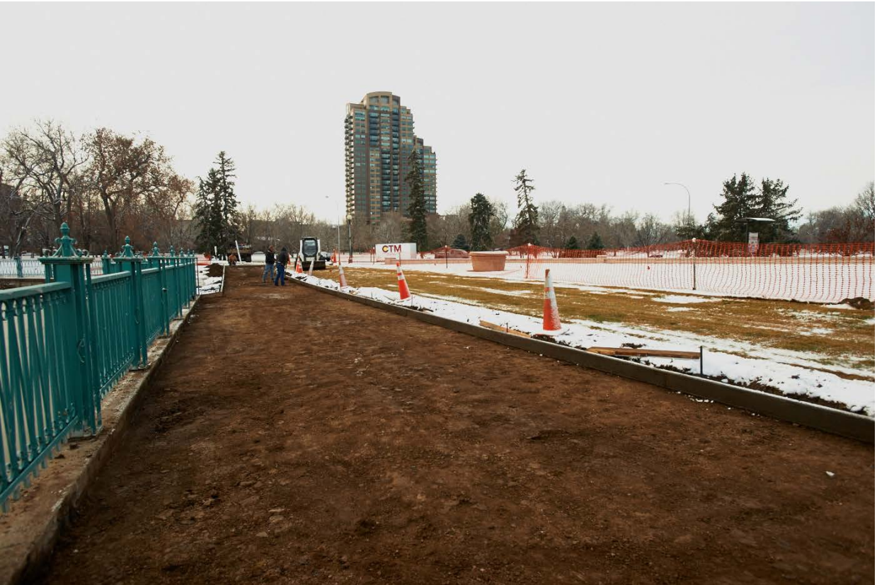
View of new roadway from Bandstand looking south.
