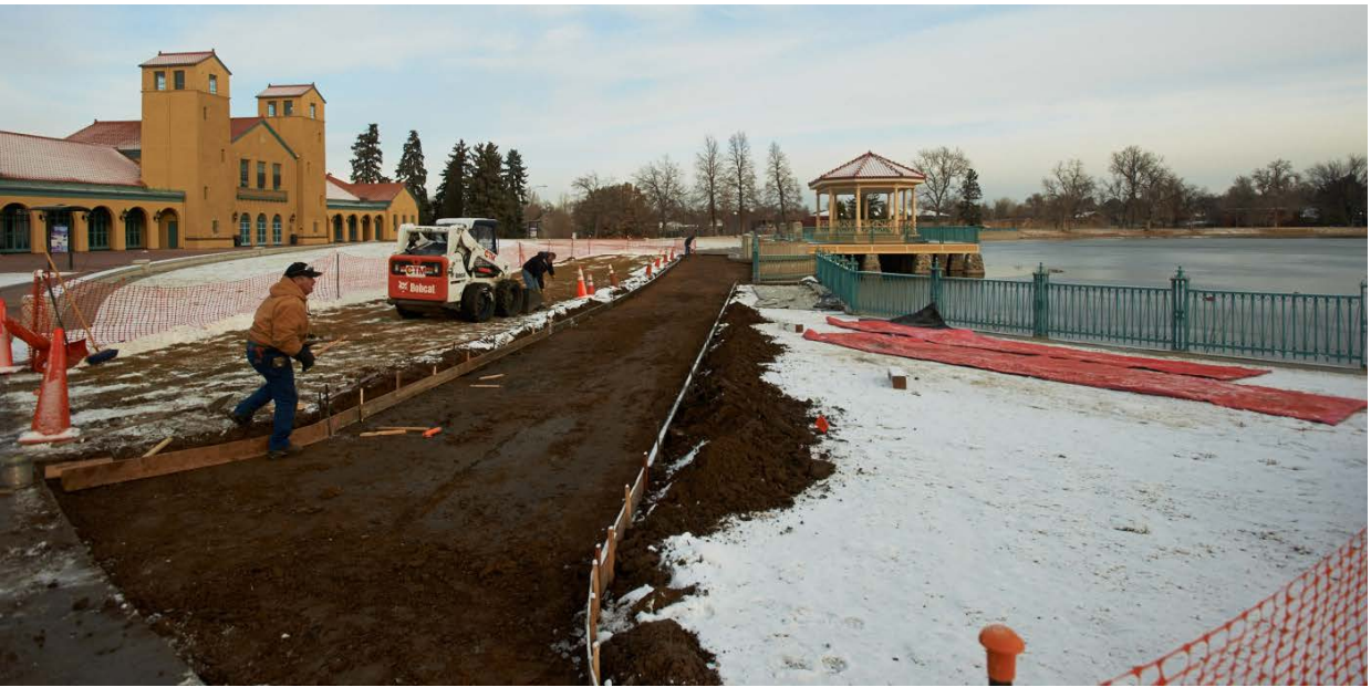
New roadway from south shore of Ferril Lake to Bandstand - December 15, 2014
