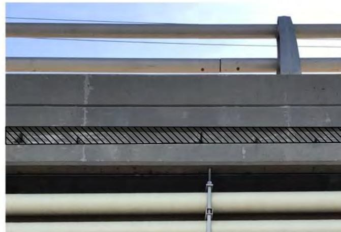
**TYPICAL INADEQUATE COVER AT NORTH FASCIA (SPAN 10) SPALL REPAIR**
