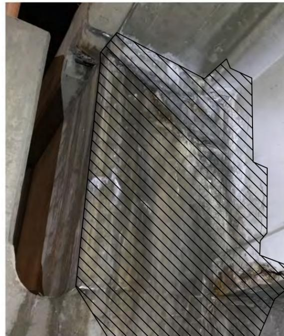
**ABUTMENT 1 - ABUTMENT AND GIRDER SPALLS**
