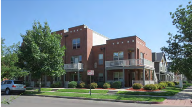
3-story walk-up apartments line 27 th Street between Lawrence and Arapahoe near the subject sites.
