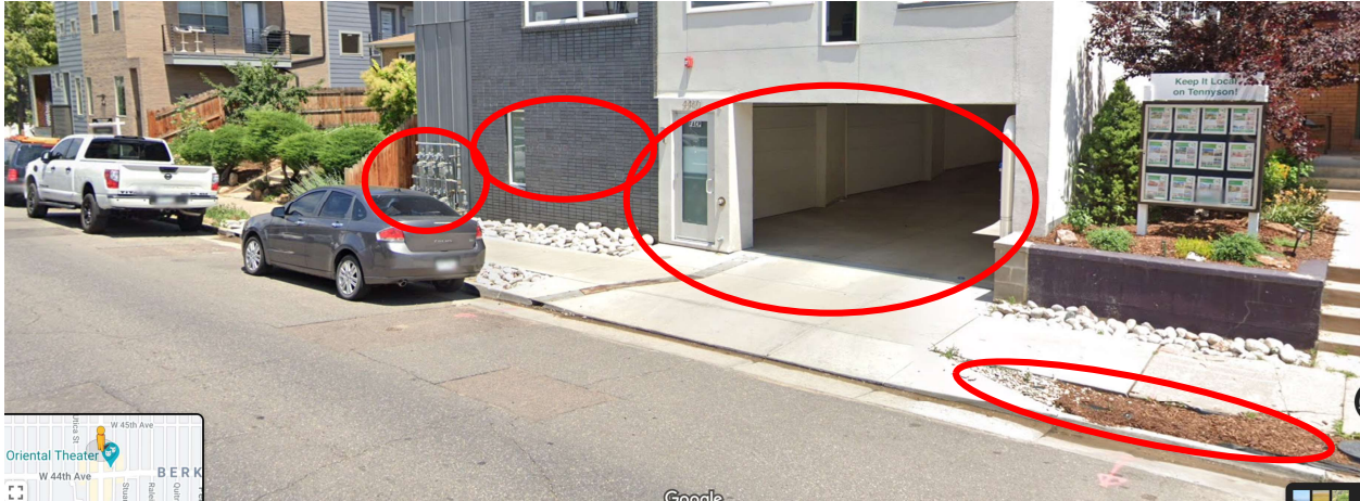
Figure 4 – Pedestrian experience includes a garage entrance, undersized tree lawn, and gas meter bank with a false front door and a single small window looking into a garage.
