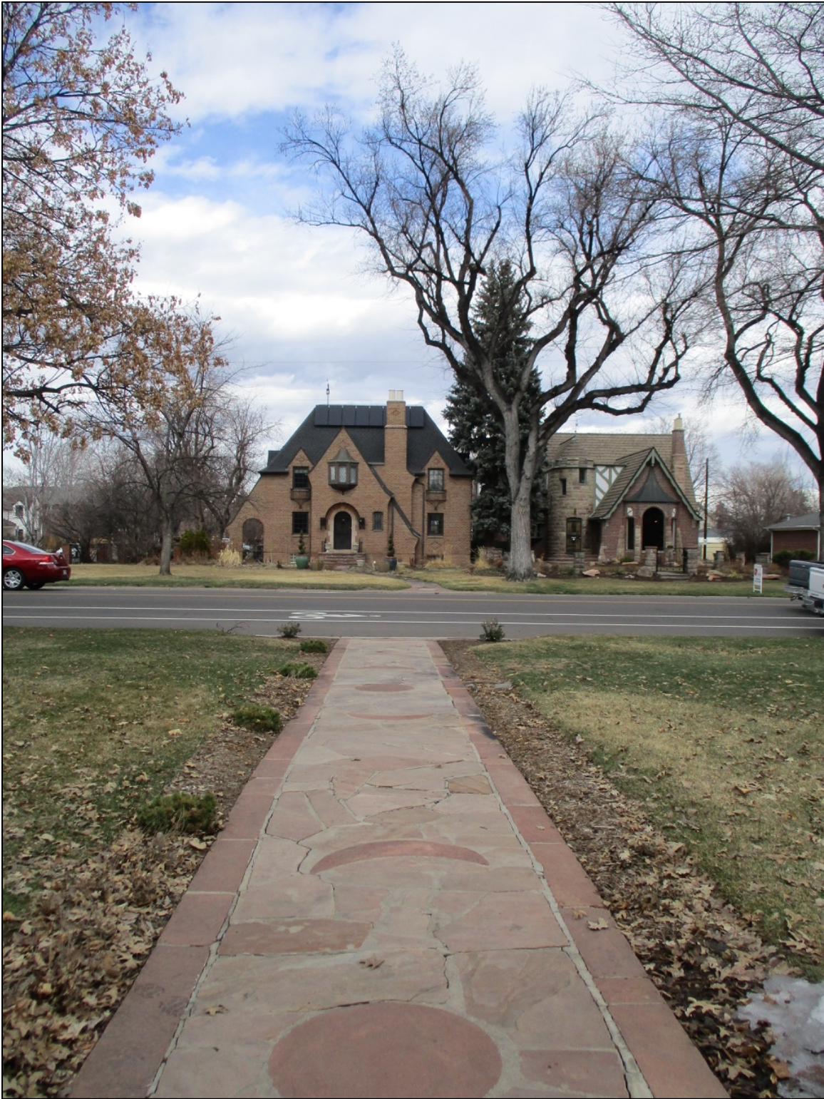
Looking north at decorative flagstone walkway. Note the decorative moon phase detail in the center.
