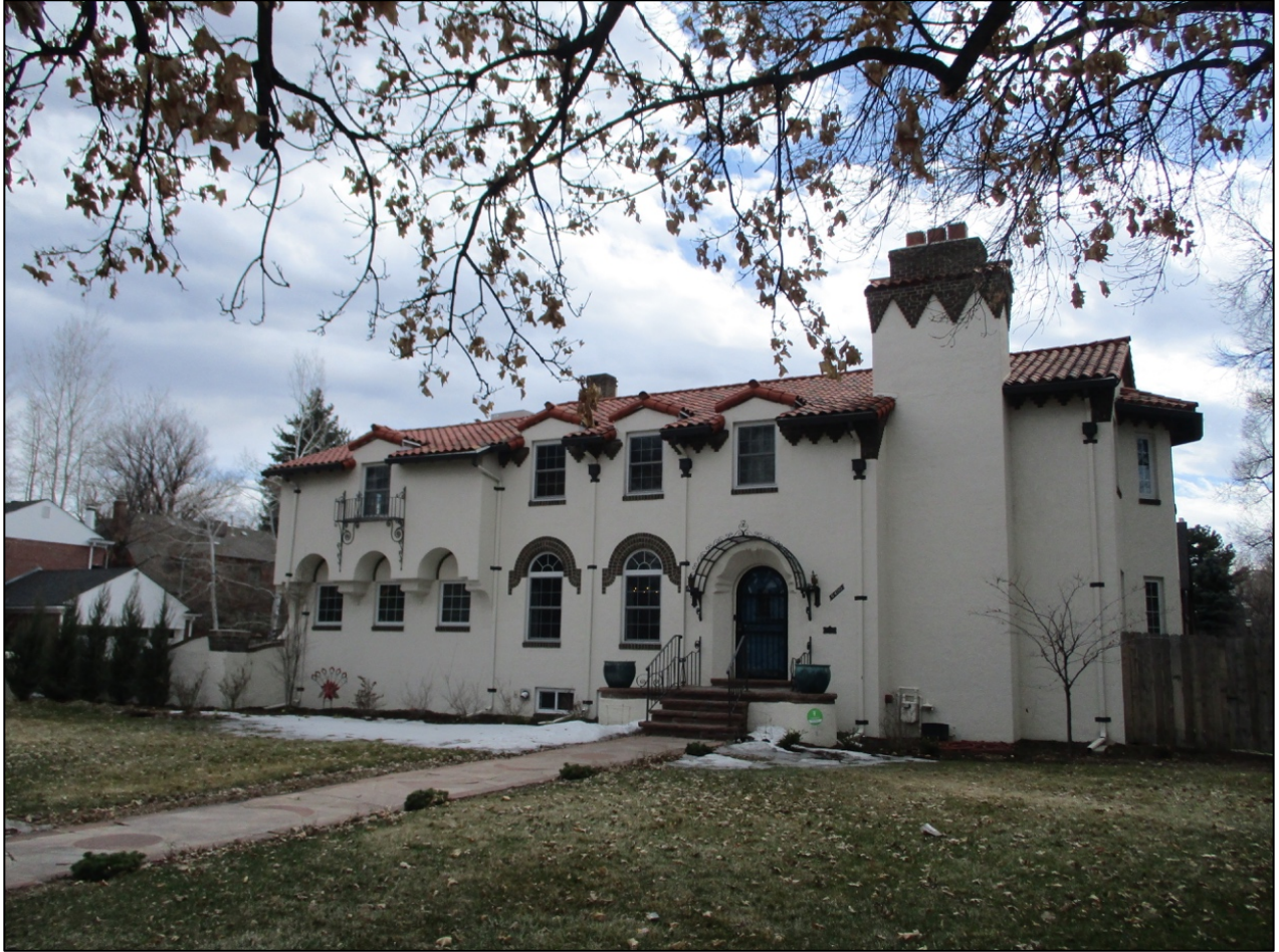
Looking southeast at north facade
