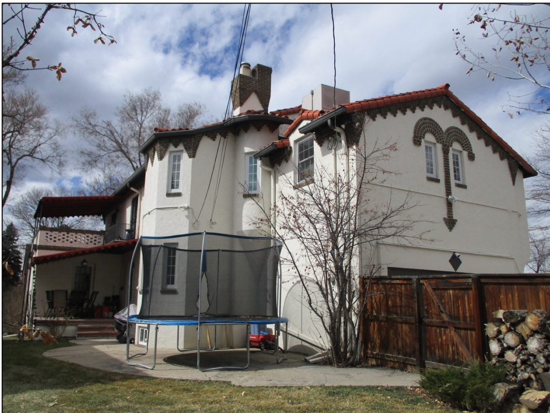
Looking northeast at west and south sides
