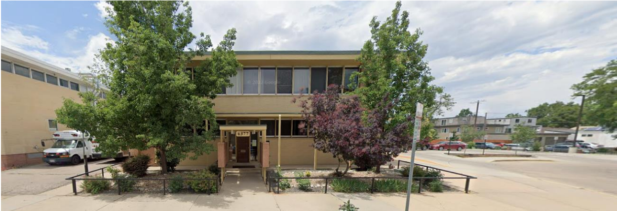
View of existing Holy Family Rectory, looking west from Utica Street.
