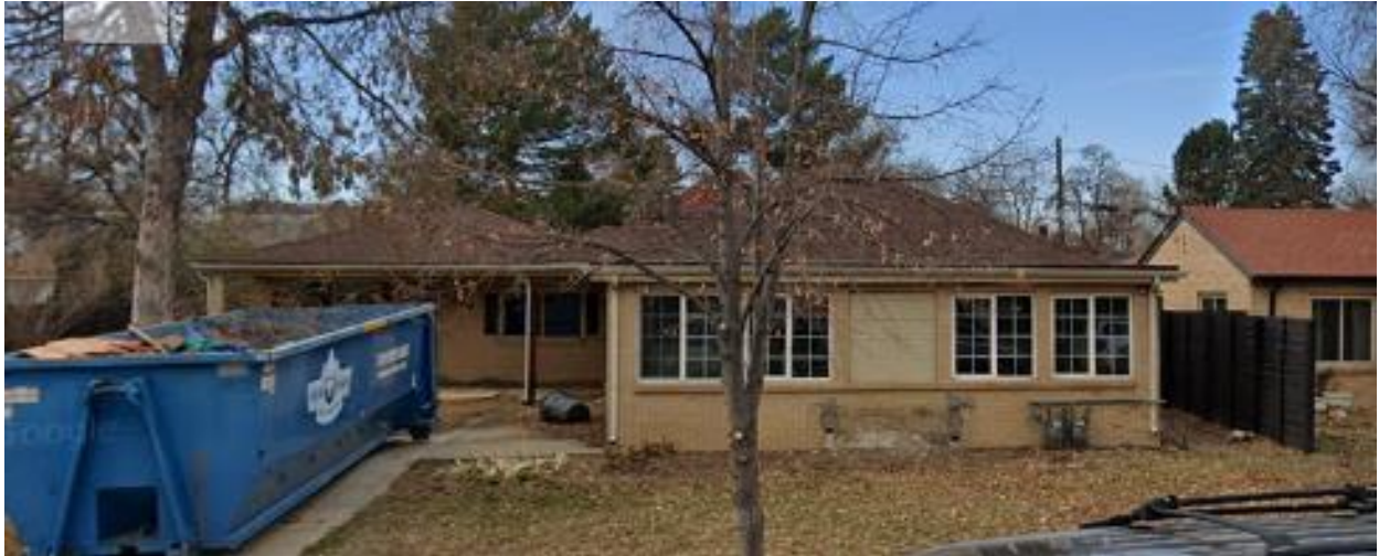
View of the property to the north, looking east.
