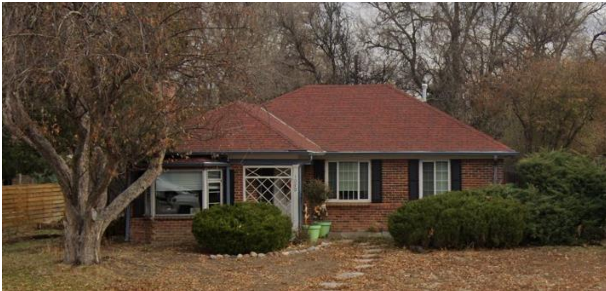
View of the property to the east.
