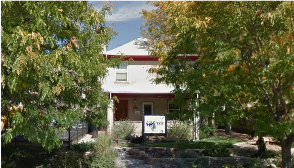
Subject property facing W 39 th Avenue
