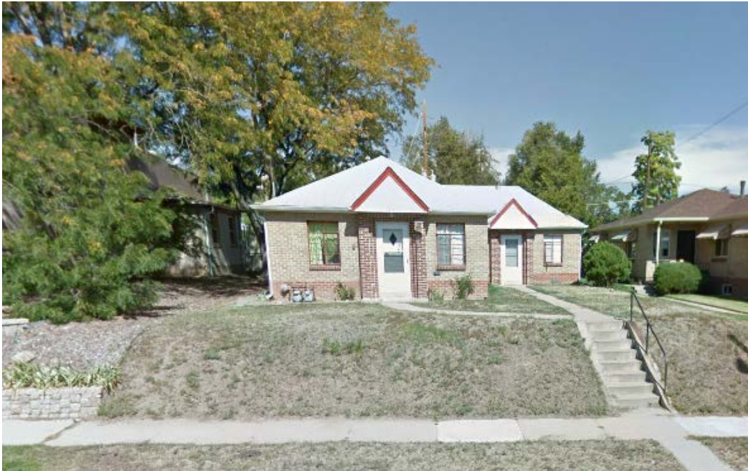
Single-story duplex directly east of the site on W 39 th Avenue
