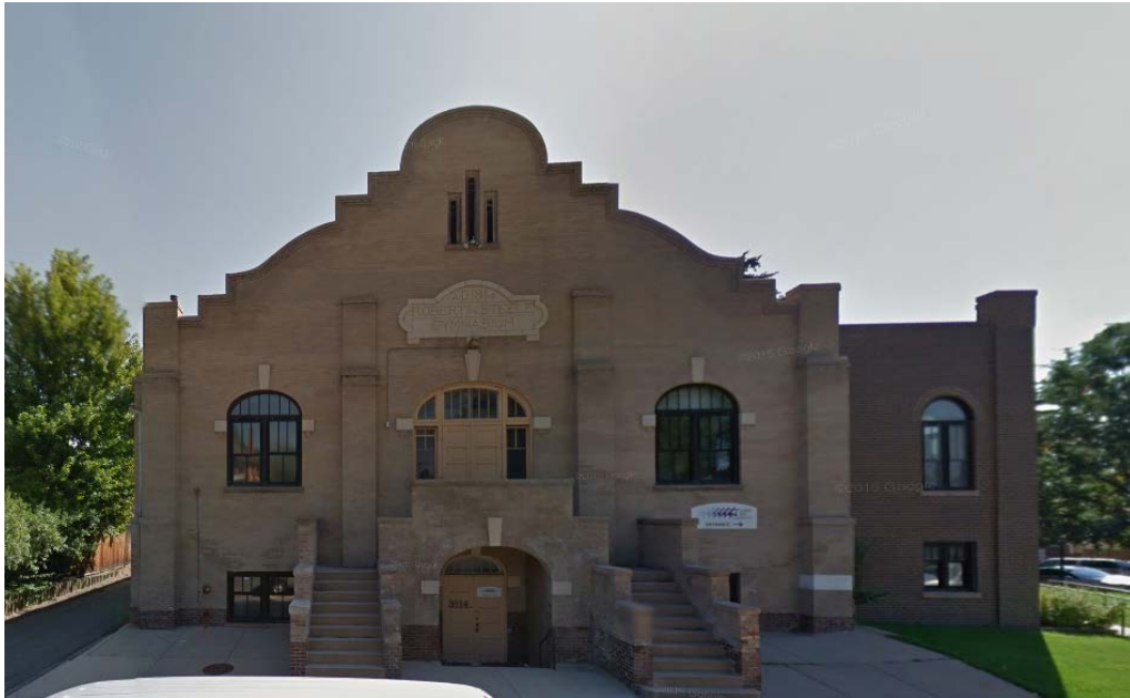
Subject property facing King Street
