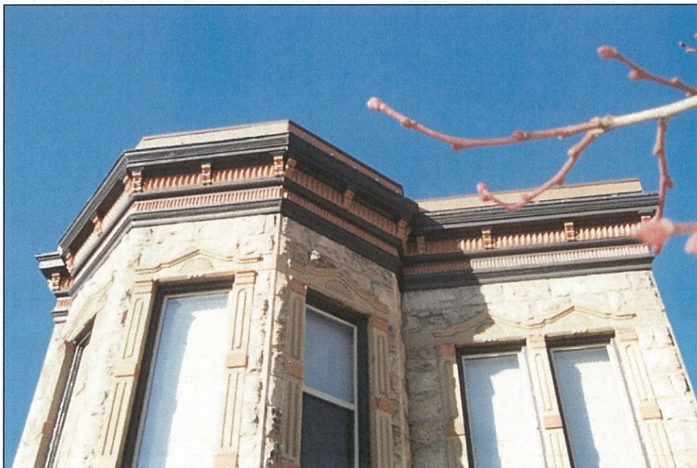
Close up of cornice at top of front façade parapet and limestone window surrounds with sandstone capitals and breaks on east side. (Photo by Patrick Salazar.)
