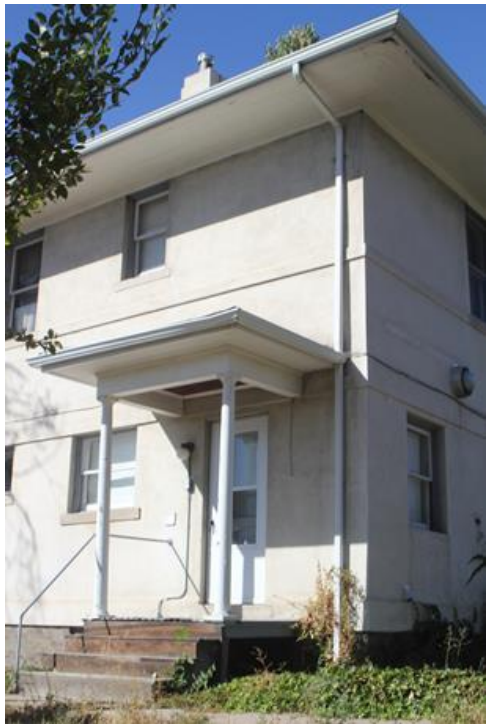
Hipped Roofed NE Entry Porch
