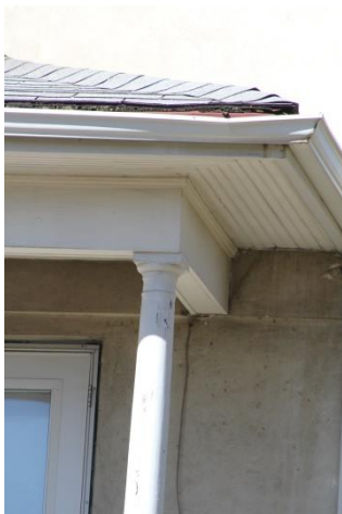
Beaded Board Eaves Soffit, Doric Column
