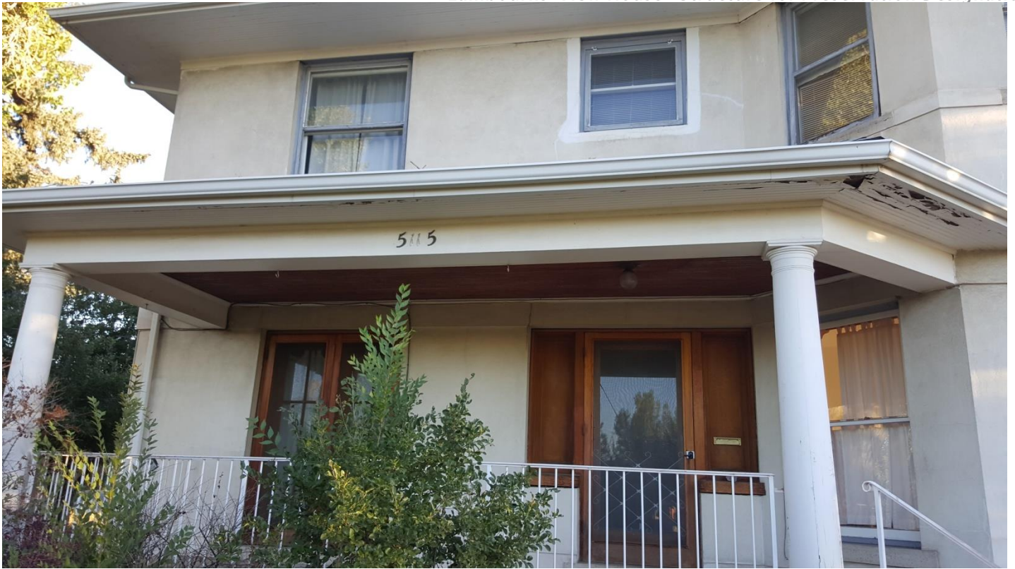
5. South Elevation Porch
