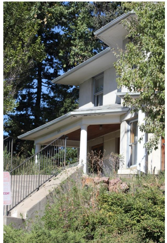
2. Top staircase to corner entrance. South Porch.
