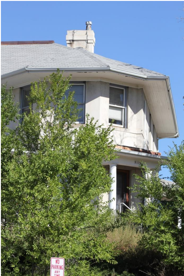
Southeast Projecting Two Story Bay
