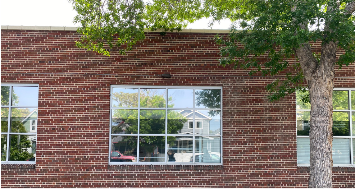
Figure 1-4 Existing West elevation showing window openings and divide light windows as well as showing fenestration pattern and solid to void ratio. Not to Scale. Illustrative Only.
