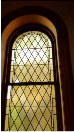
Original stained glass window
