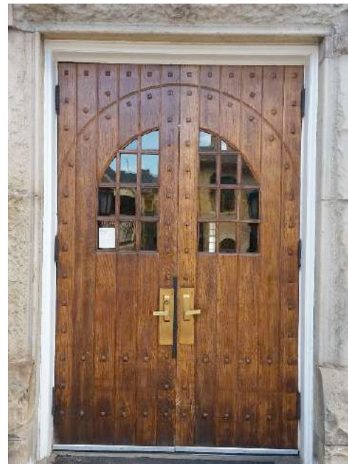
Original doors that remain on building
