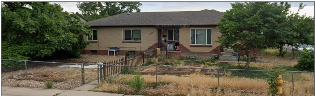
View of the property to the west (across the alley), looking east on N. Locust St.
