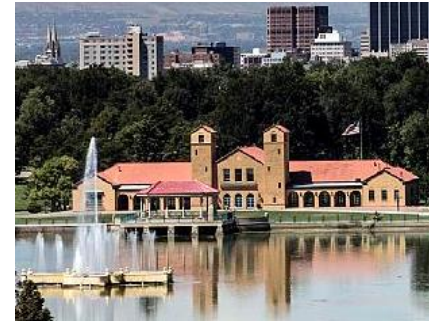
City Park Pavilion
