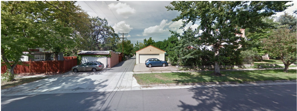
View of the property to the west (other side of the alley), looking north.
