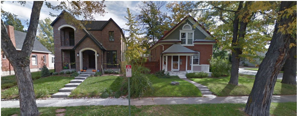
View of the property to the north, looking east.
