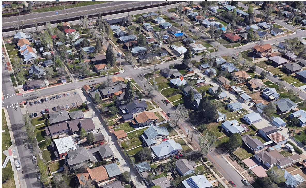
Aerial view of the site.
