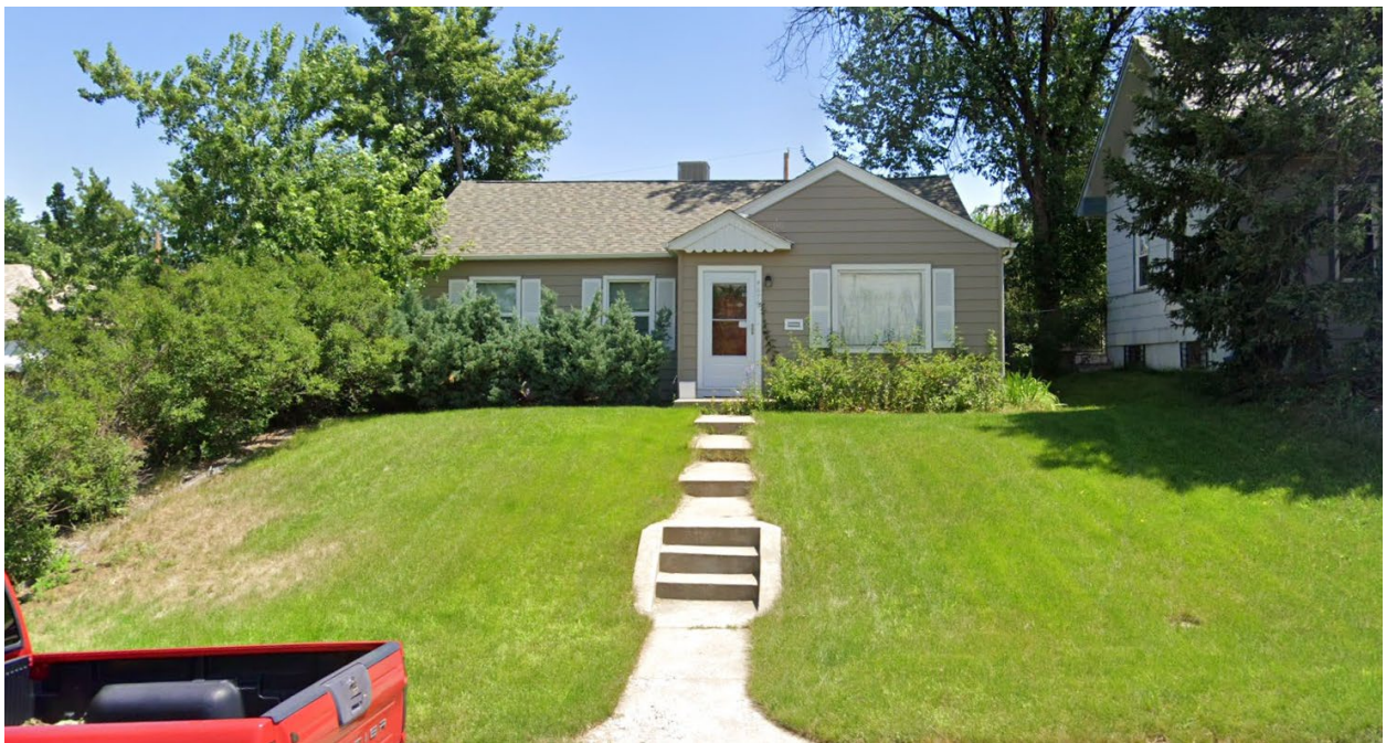
View of the property to the south, looking east.
