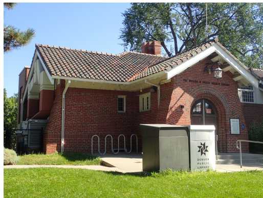
6: Smiley Branch Library. Note materials and impact of roof tiles
