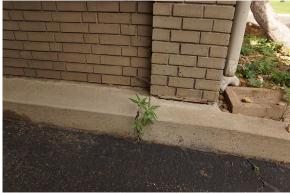
4050: Cracked concrete
