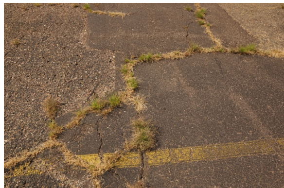
4031: Cracked/weed-filled asphalt
