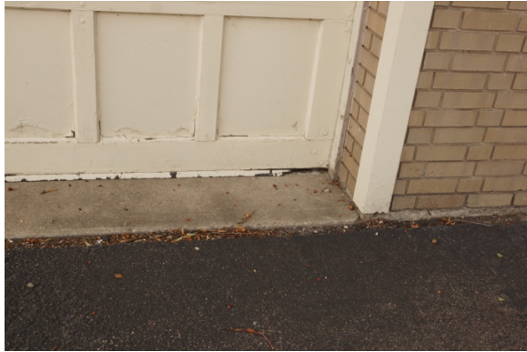
4026: Garage door ground movement
