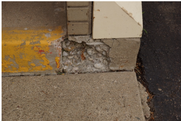
4024: Concrete spalling
