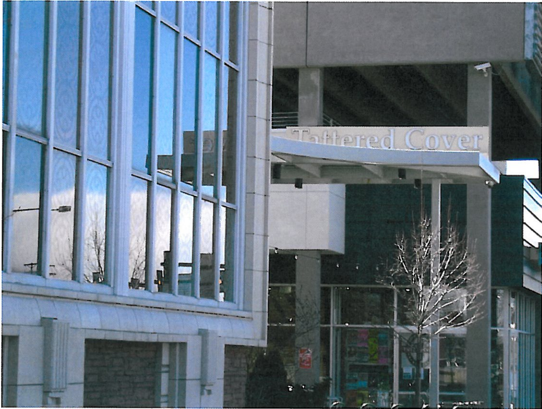
Aluminum Canopy with new Tattered Cover Signage
