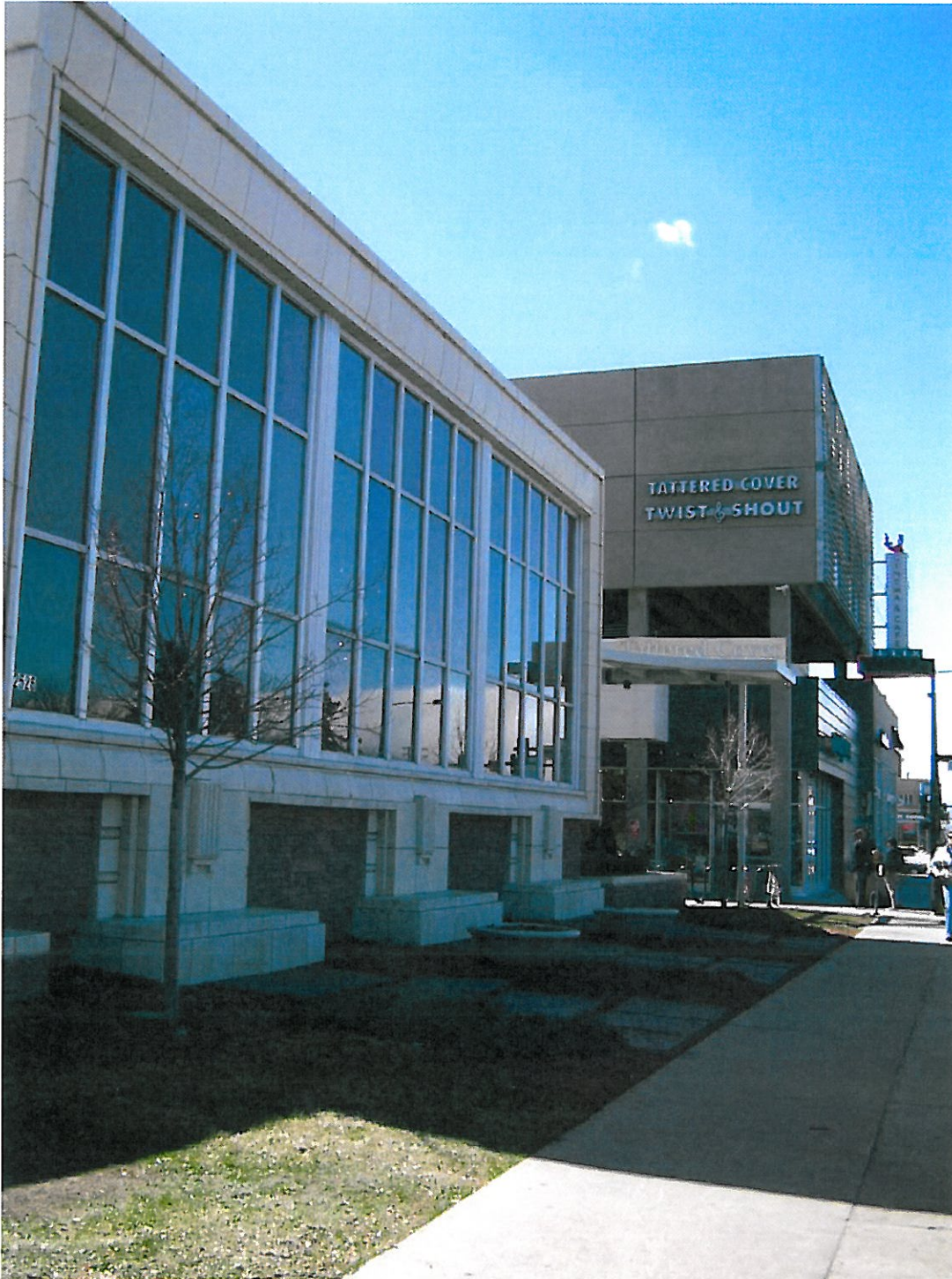
Colfax Avenue Façade- This acts as the main façade for the new bookstore. A new canopy with bookstore signage was installed. The original rose colored windows with circle motif were retained.
