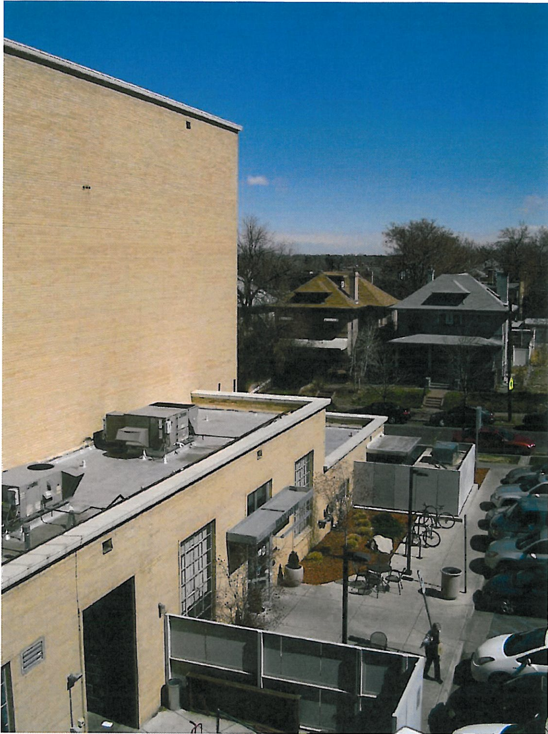
South Façade- This façade is dominated by the towering fly-loft structure. An auxiliary entrance is flanked on either side by a loading bay and screened building service components.
