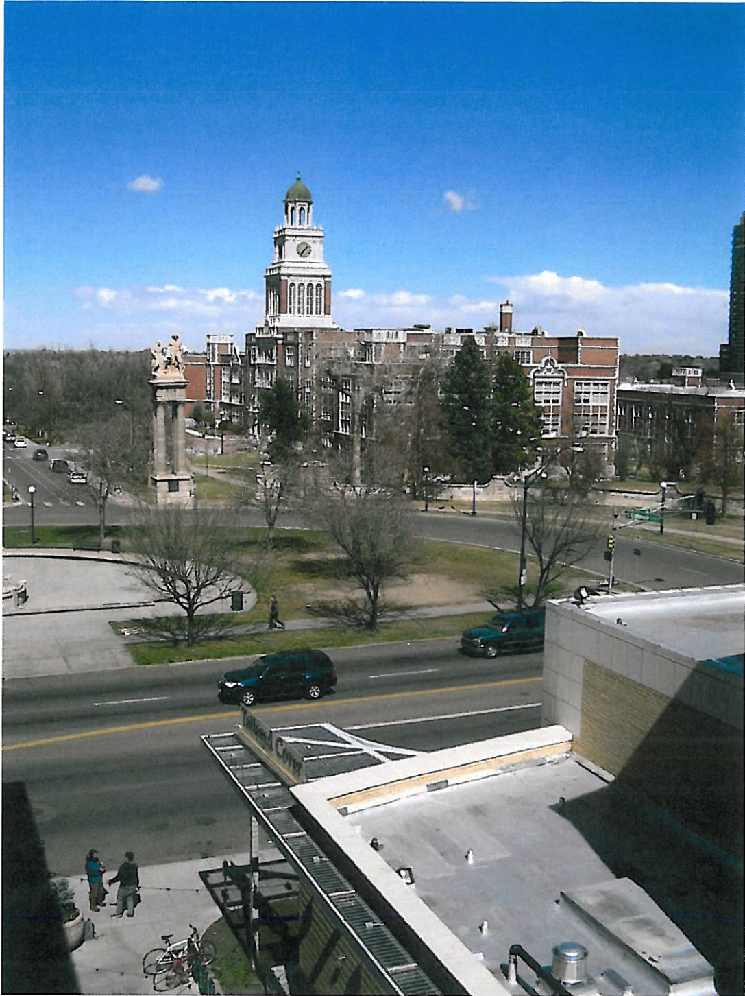
A pedestrian walkway separates the Lowenstein Theater building from the adjacent parking structure. Across Colfax Avenue are the Sullivan Gateway and East High School, other historic structures.
