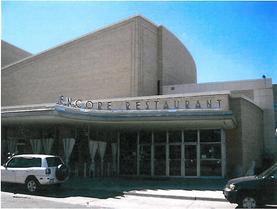
Elizabeth Street Façade- The former theater ticket foyer was converted into the space for the Encore Restaurant.
