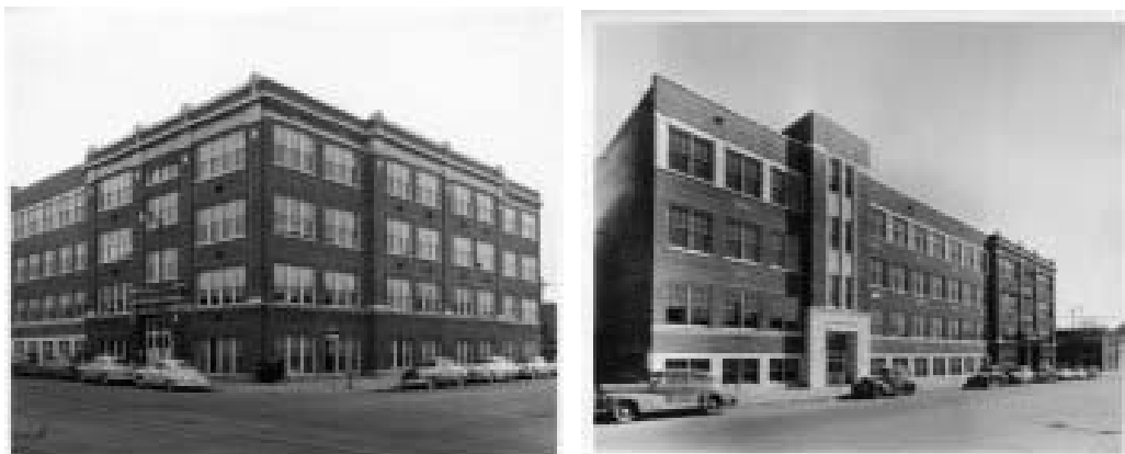
Historic photograph of the 1926 Addition on left (1941) and the 1947 Addition on right (1949), Courtesy Denver Public Library
