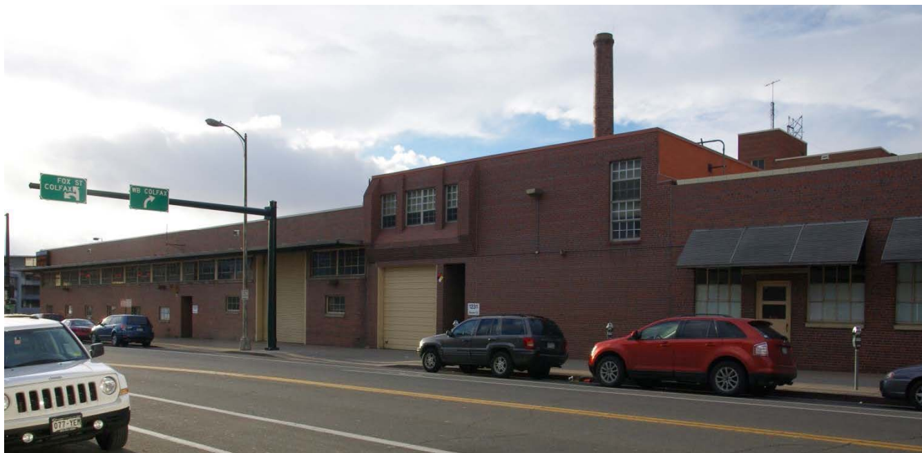
Photo, from left to right, of the 1954 Body Shop, the 1978 Auto Shop and the 1941 Shop Building on Glenarm Place. These accessory structures are located in the Non-Contributing Area of the designation.
