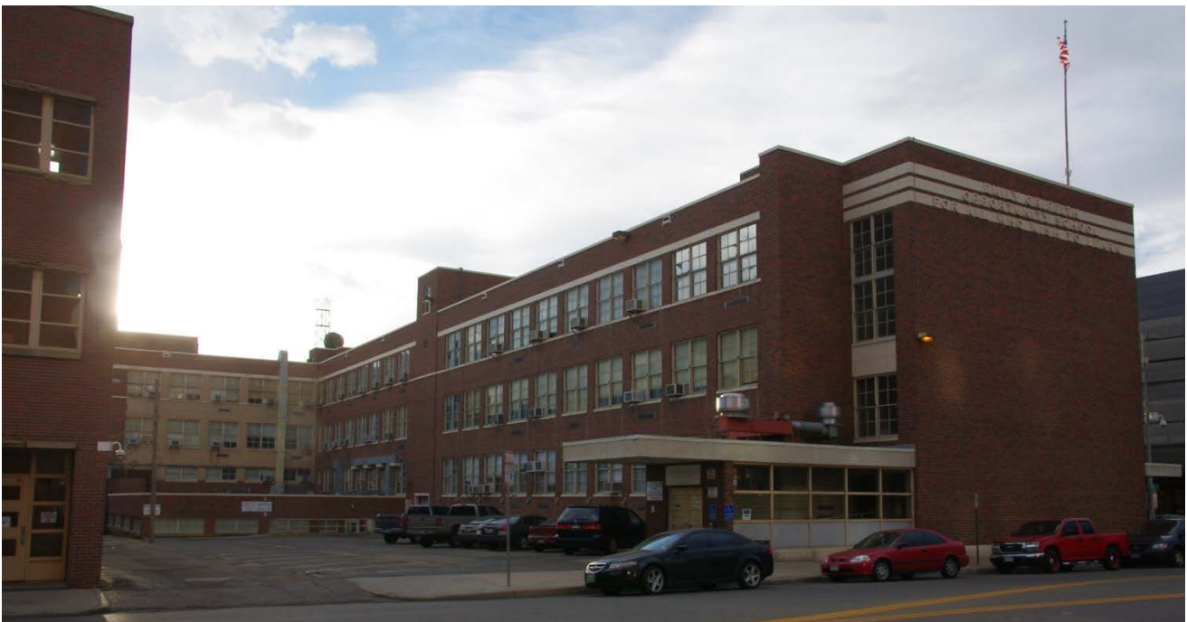
View looking northwest at the rear of the 1956 addition and its entry vestibule from 13 th Street
