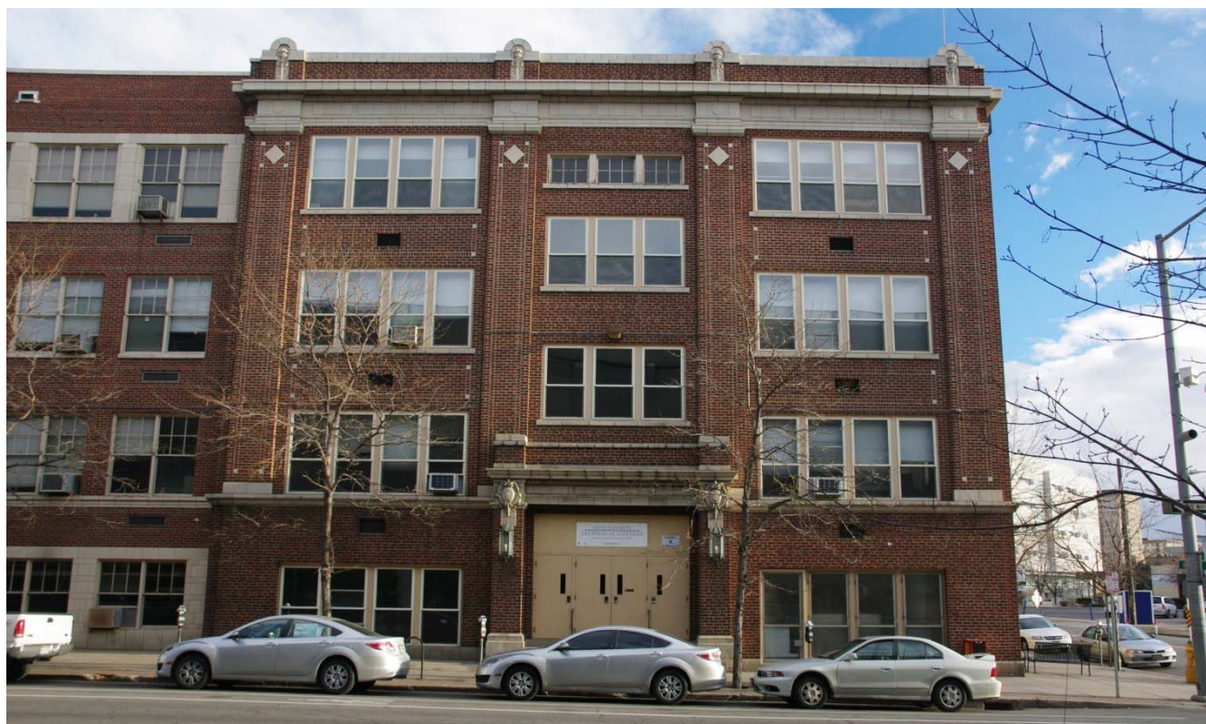
View of the Welton Street façade of the 1926 Opportunity School Building. This is the earliest building on the site and the only one dating from Emily Griffith's tenure at the School.
