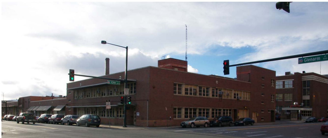
The 1956 KRMA Building, located on the corner of Glenarm Place and 13 th Street. This structure would be considered Non-Contributing to the Landmark designation.
