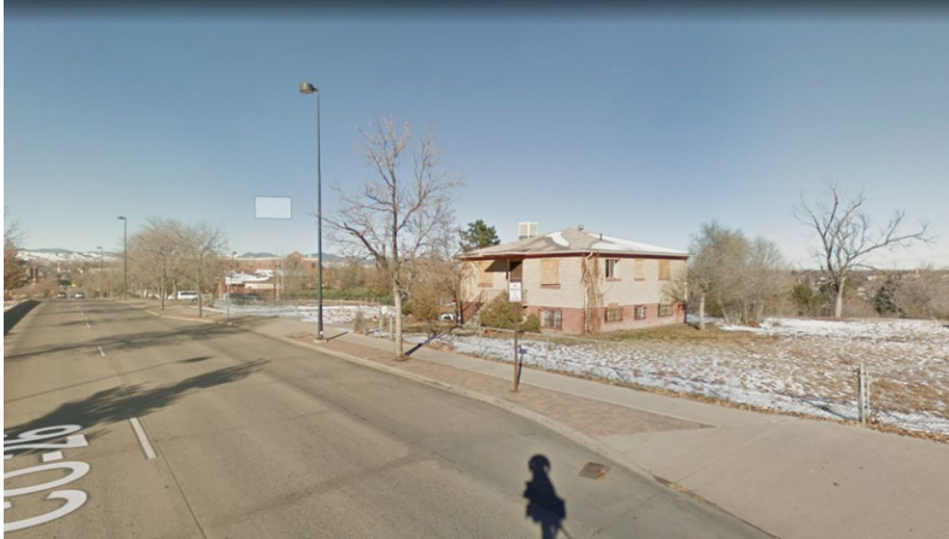
Subject property, from W Alameda Avenue (single-unit residence)
