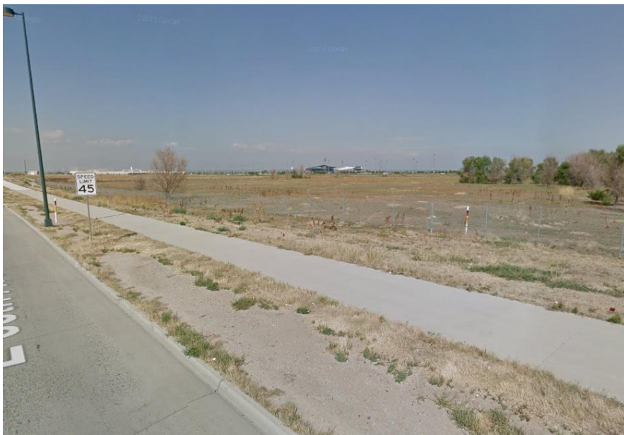
56 th Avenue looking northwest from subject site
