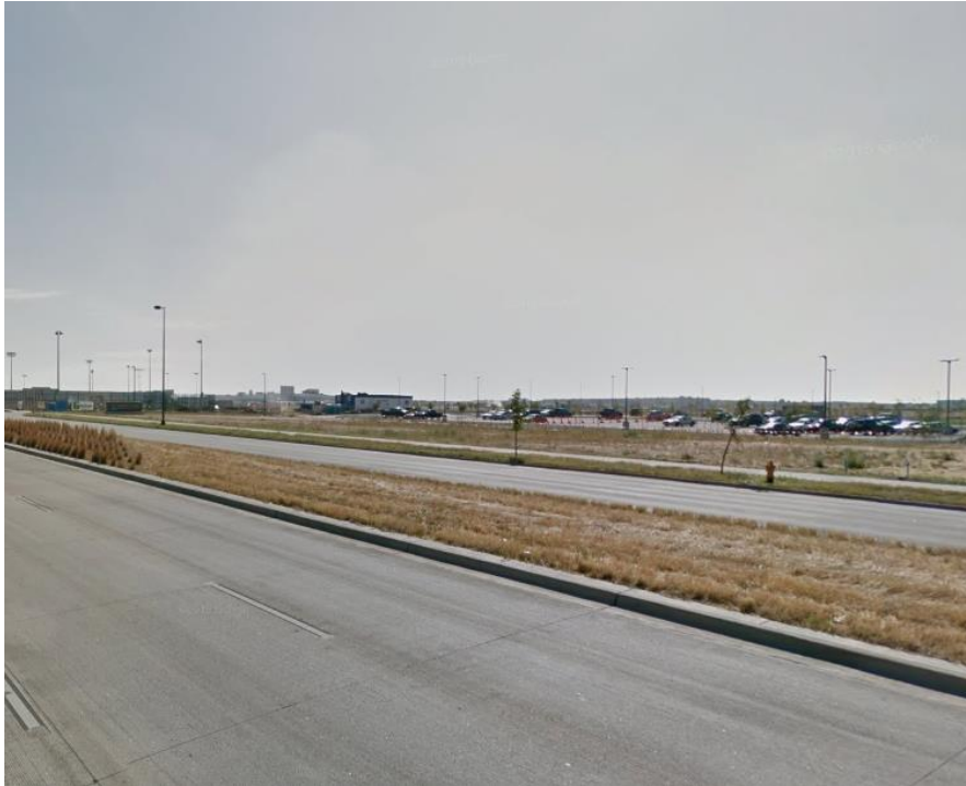
56 th Avenue looking southeast from subject site
