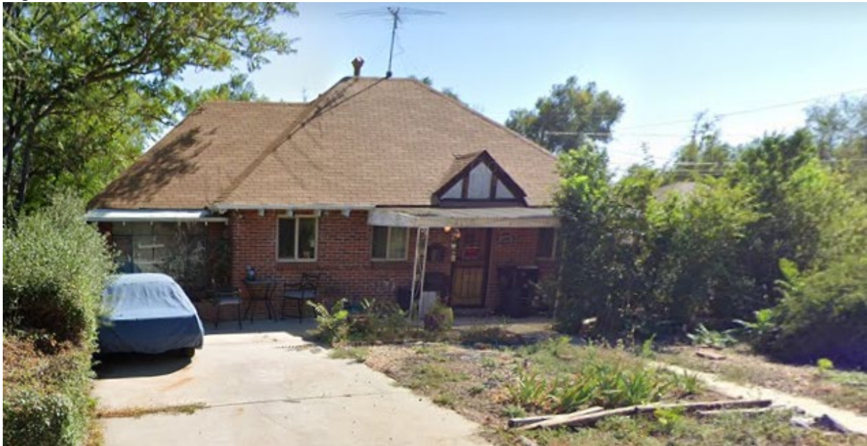
View of the property to the north, looking east.
