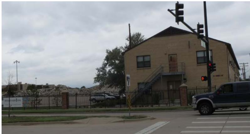
4 Vacant property south of subject property
