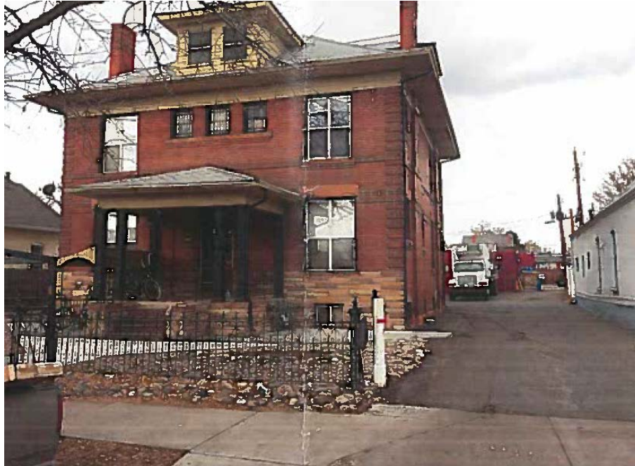
View of the Remaining Building defined in PUD-G 16 from Tejon Street looking west showing existing drive aisle on north side of subject property.
