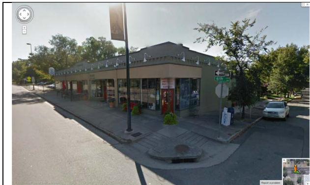
View looking southeast from 6 th Avenue & Gilpin Street
