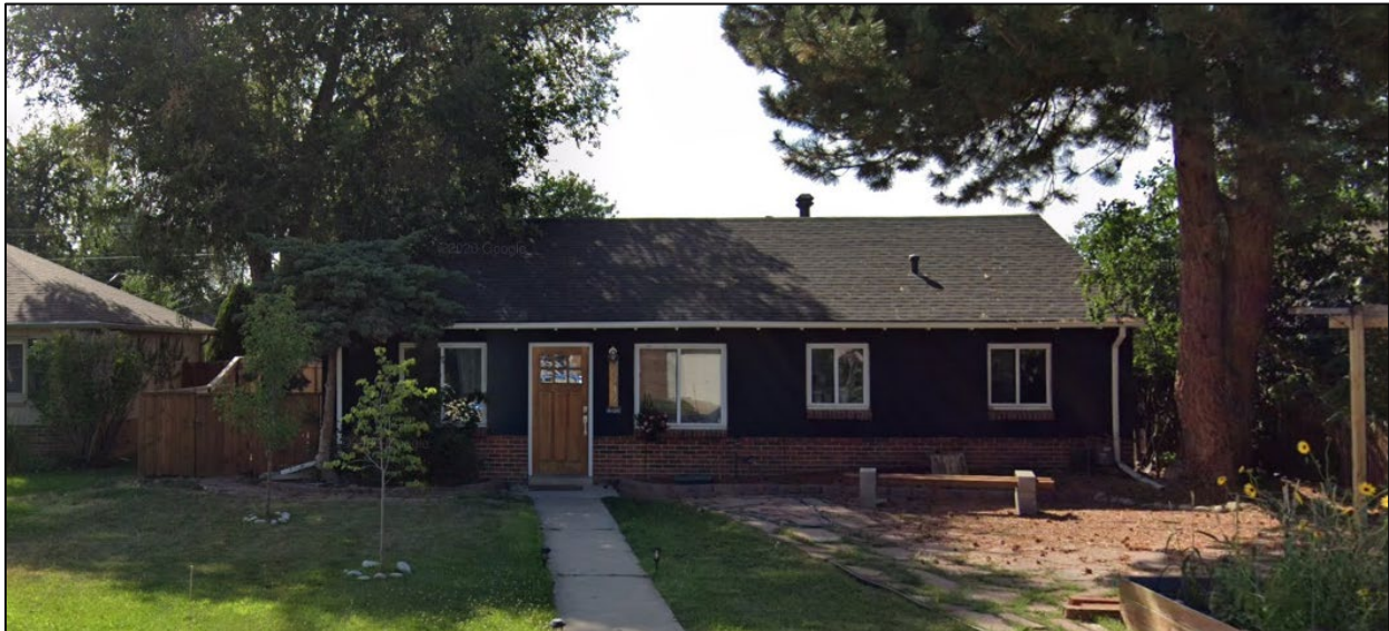
View of the subject property looking west.
