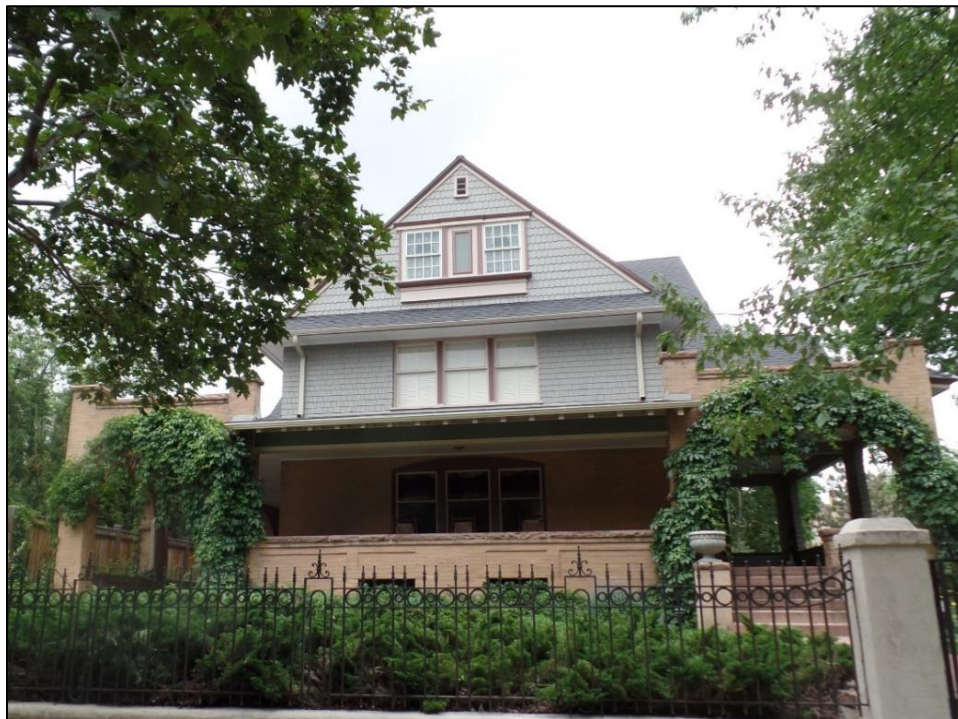
670 Marion Street, front façade
