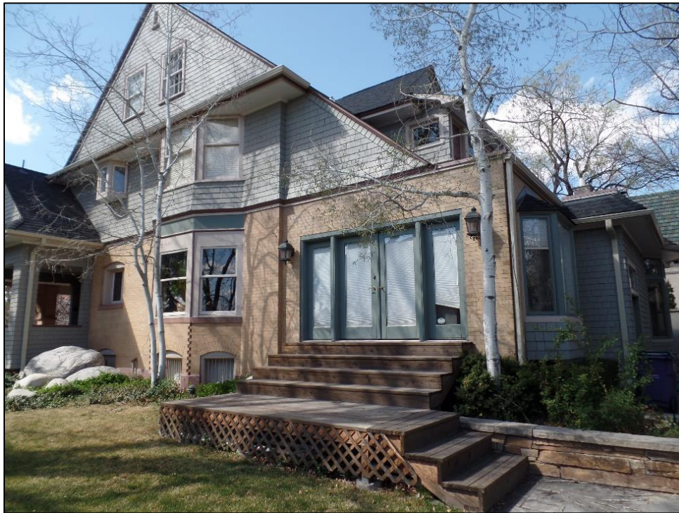
670 Marion Street, side and rear elevations
