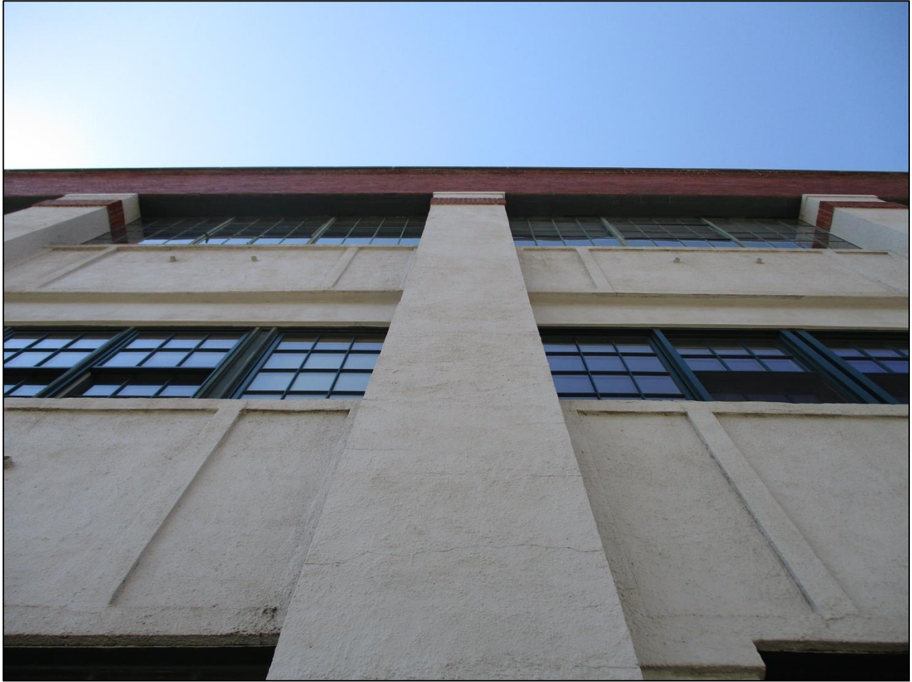
Looking up at north façade exterior
