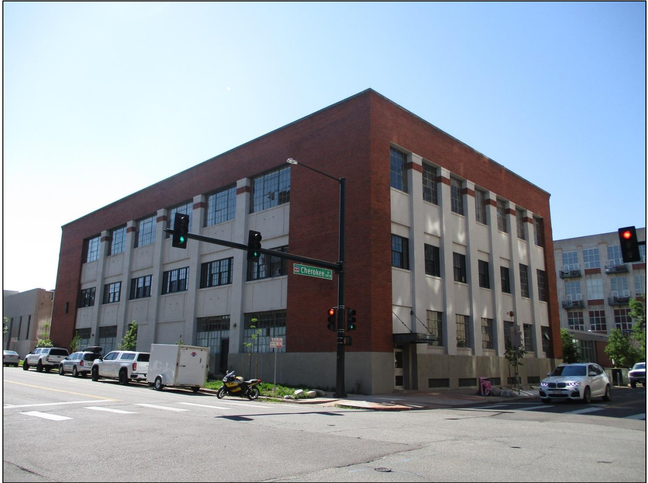
Looking southeast at west and north façades
