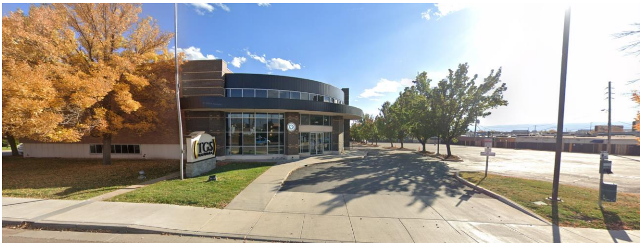
View of the subject property from Arkansas Avenue, looking south (Source: Google Maps)
