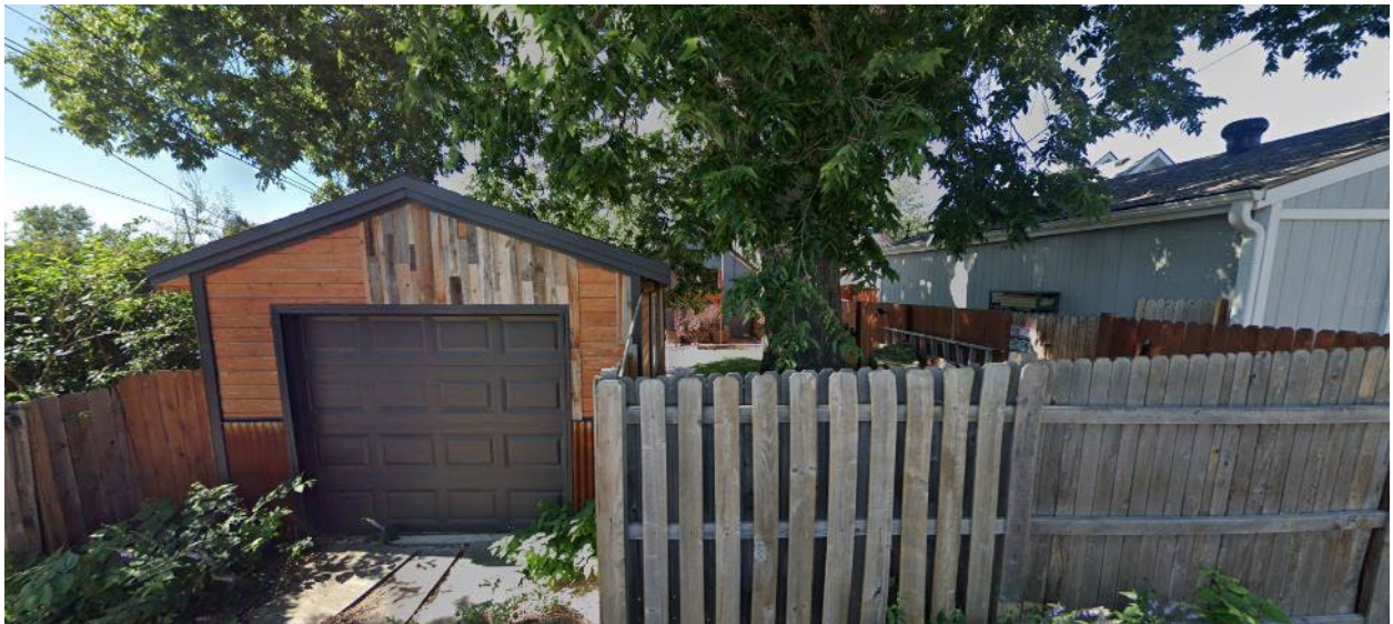
View of the subject property's garage, looking south from the alley.
