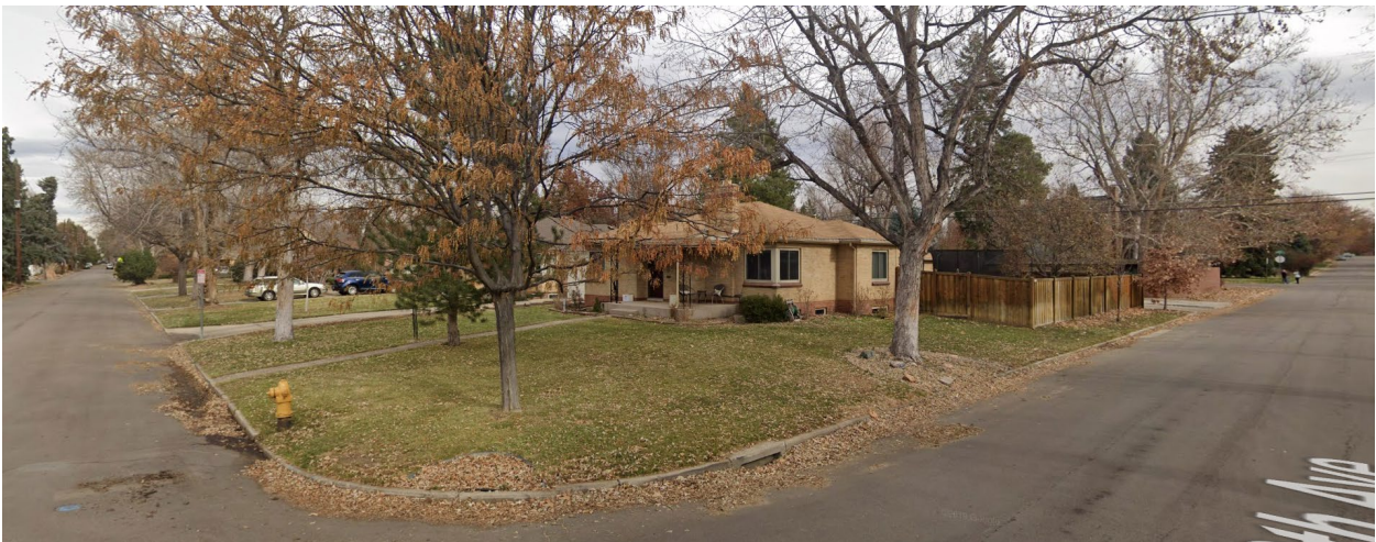
East - View of the property to the east (across from North Magnolia Street), looking northeast.
