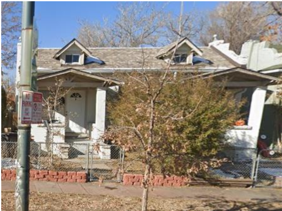
View of the property to the north, looking west.
