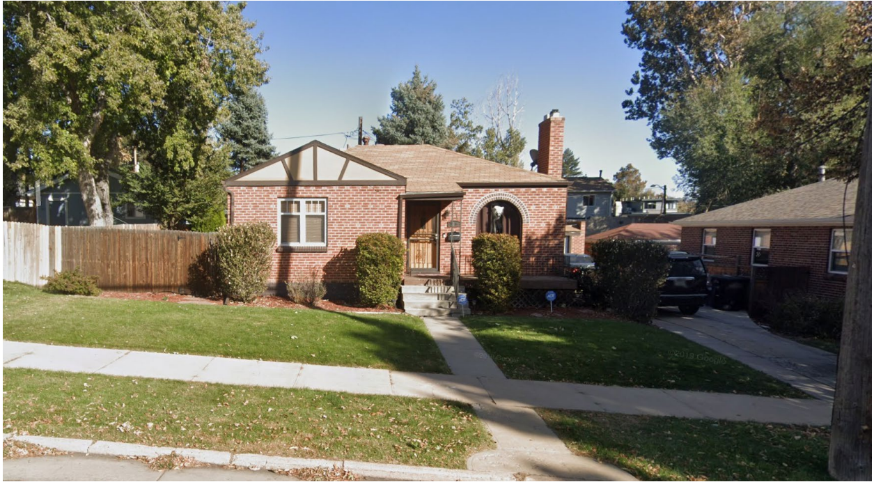
View of the property to the east.
