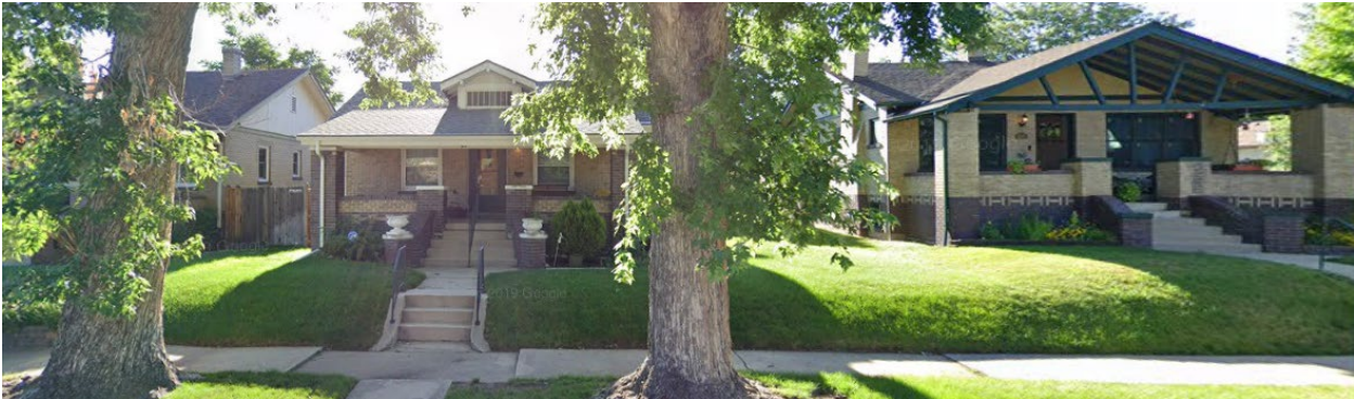
View facing east on Knox Court north of 42 nd Avenue – within proposed rezoning
