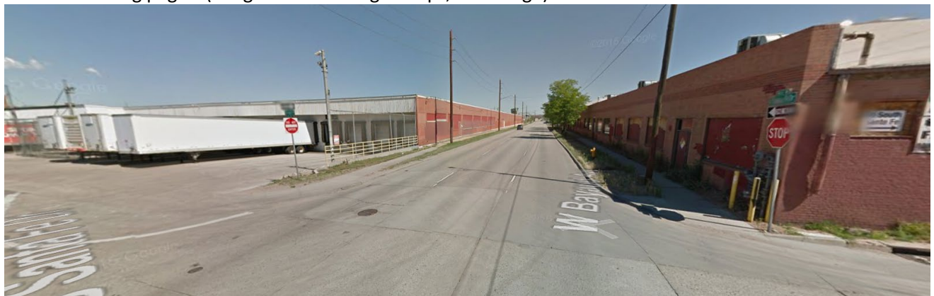
View of 50 S. Kalamath St. (subject site - left) from the intersection of S. Santa Fe Dr. and W. Bayaud Ave., looking north.
