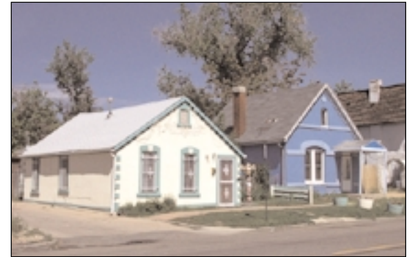
Appropriate roof pitch and orientation
