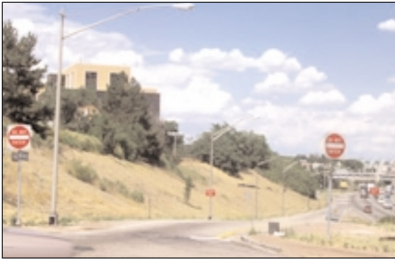
Site of slip ramp and promenade
