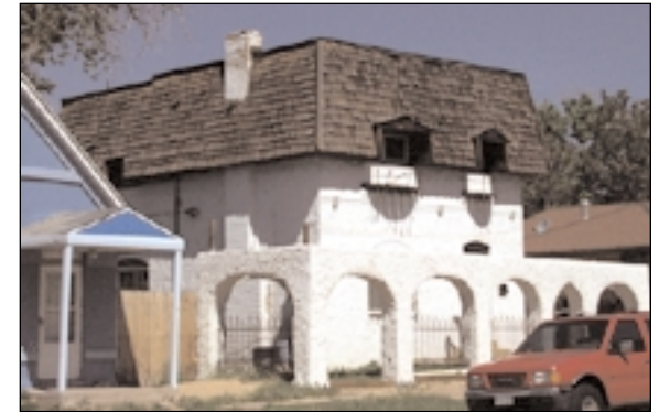
Inappropriate window orientation
