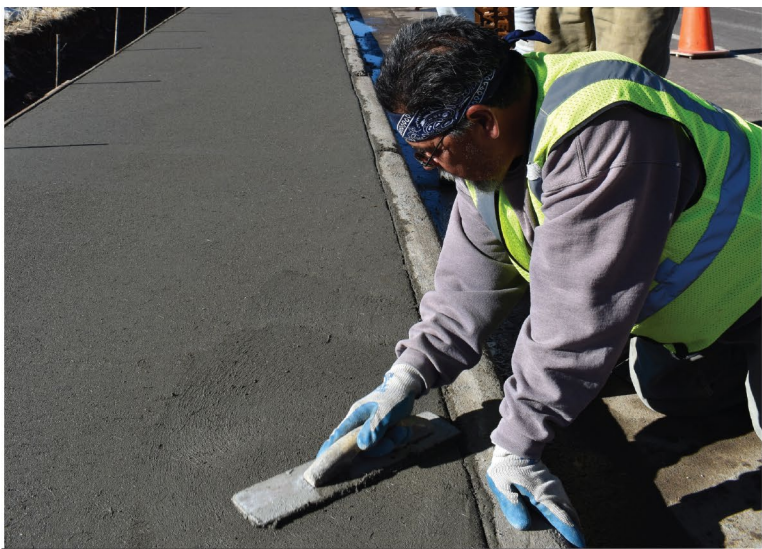
W Dartmouth Ave. - First Sidewalk Paving
