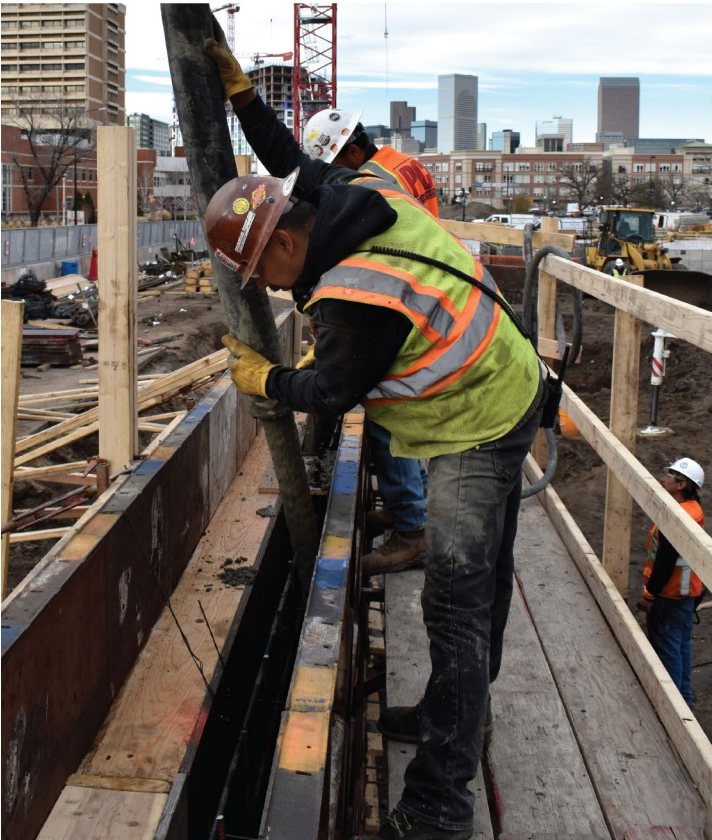
Denver Health - Poured foundation for the new OMC
