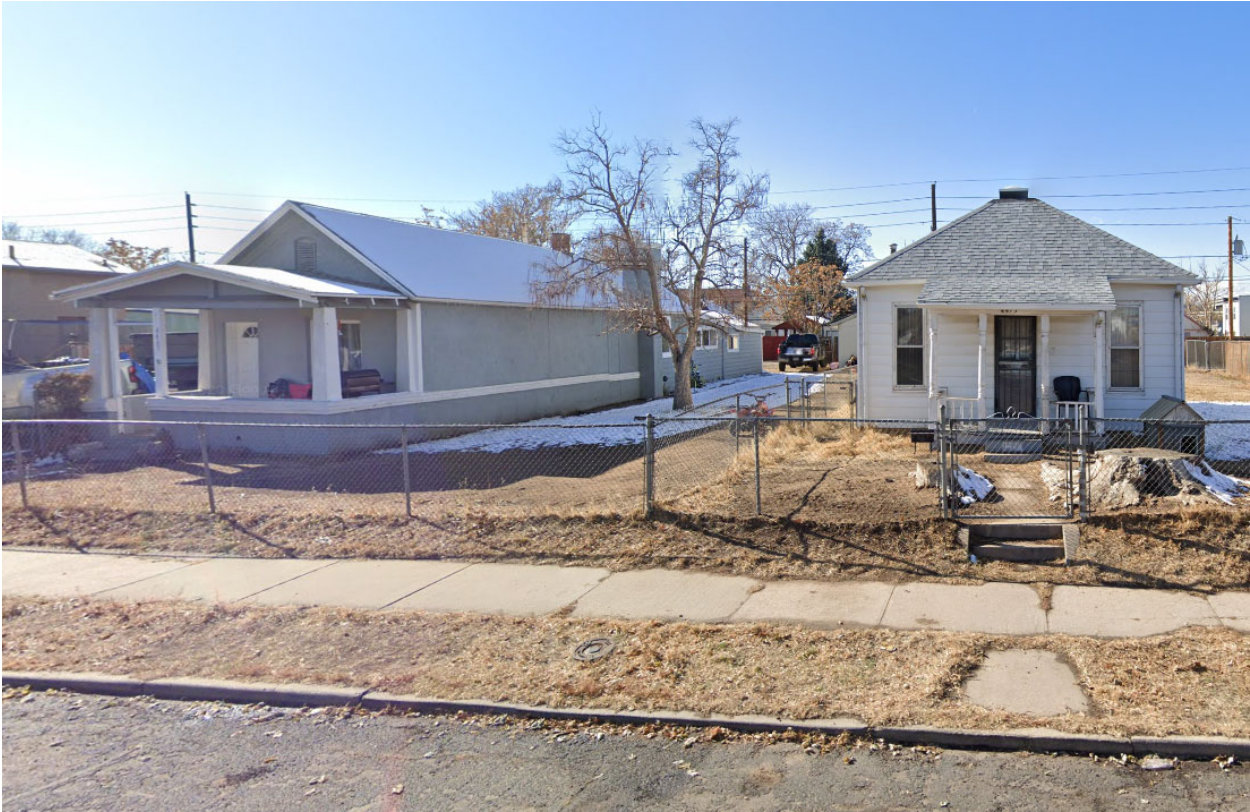
East - View of the properties to the east across North Grant Street.
