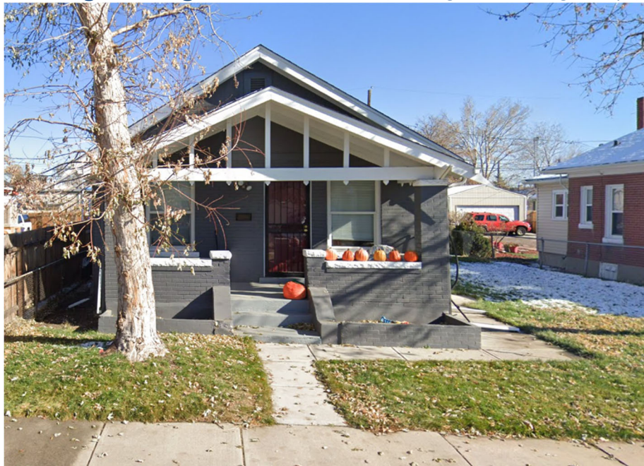
Subject Site - View of the subject property, looking west.
