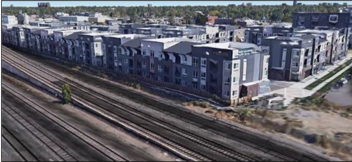
Photo 4-1. Encore Evans Station Apartment Complex
