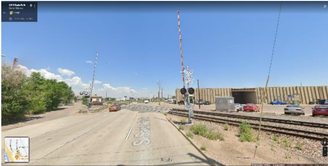
Photo C-3. South Santa Fe Drive Crossing
