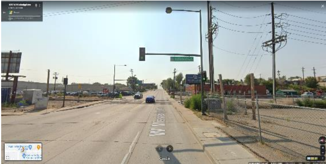
Photo C-8. West Mississippi Avenue Crossing
