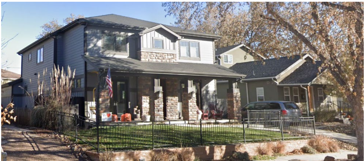
South - View of the properties to the south, looking east.
