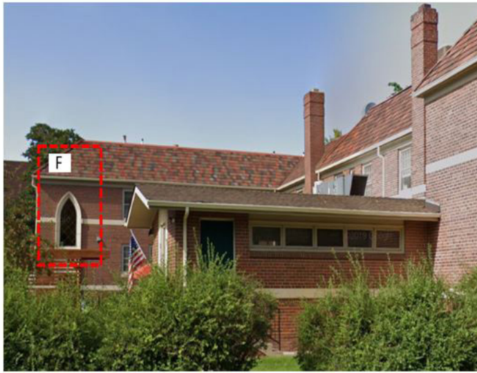
Figure 1-4: Facade Feature F
