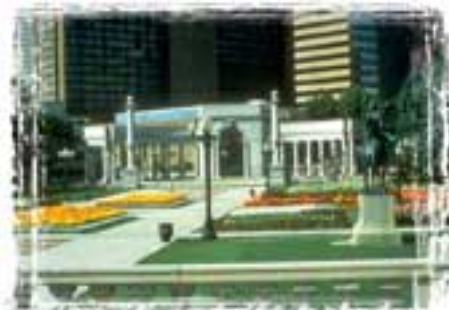
Voorhies Memorial sits at one end of the promenade in Civic Center Park
