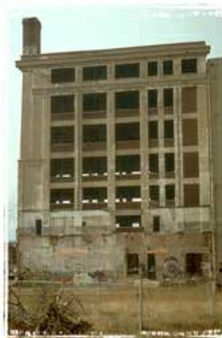
A long-vacant flour mill under renovation to lofts in the Central Platte Valley
