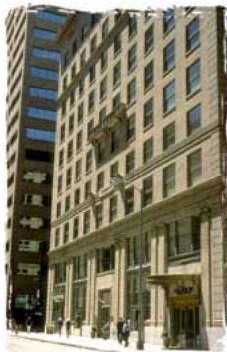
The Guaranty Bank Building on 17th Street, prior to its renovation
