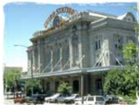
Union Station is a historic anchor for Lower Downtown
