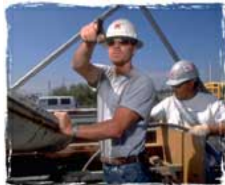
Upgrading our infrastructure: construction on Speer Boulevard Bridge
