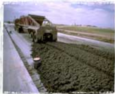
Roadway construction to support growth
