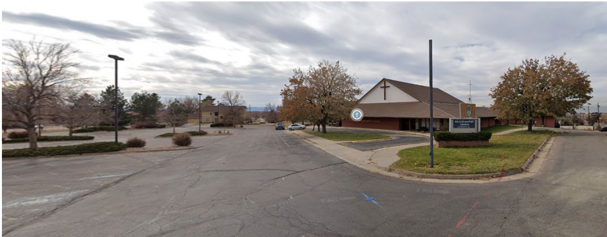
Site - Looking west from the parking lot
