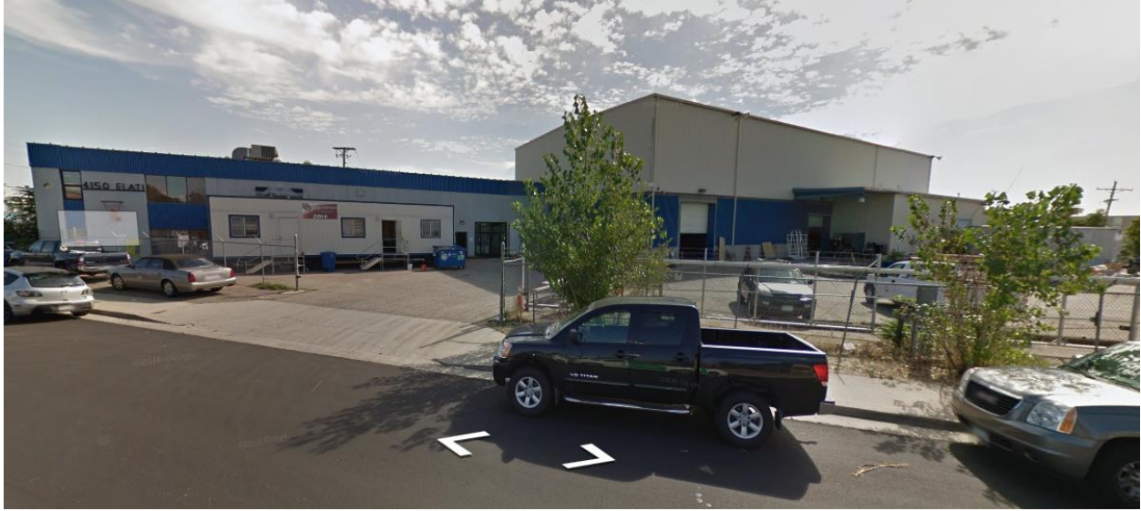
Two-story industrial structure to the north, looking northeast.
