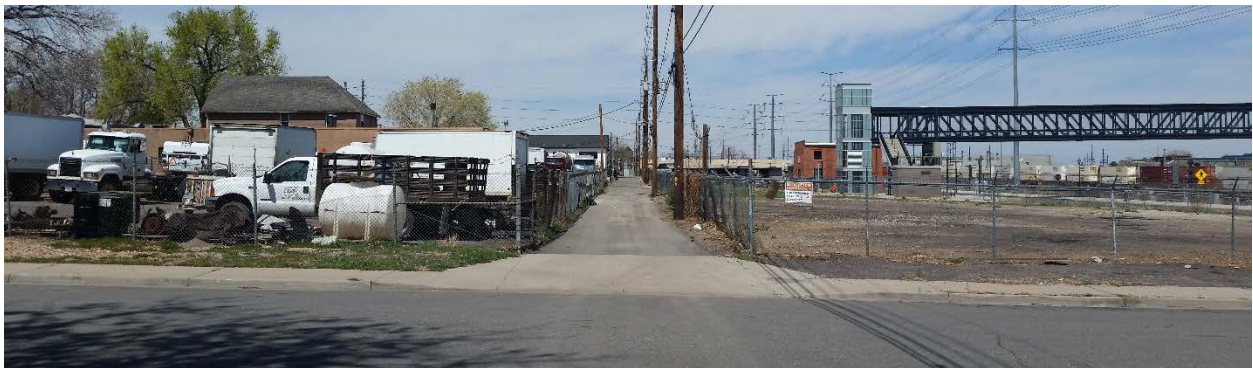
View of the site looking north from 40 th Avenue, with the public alley that bisects the properties running north/south
