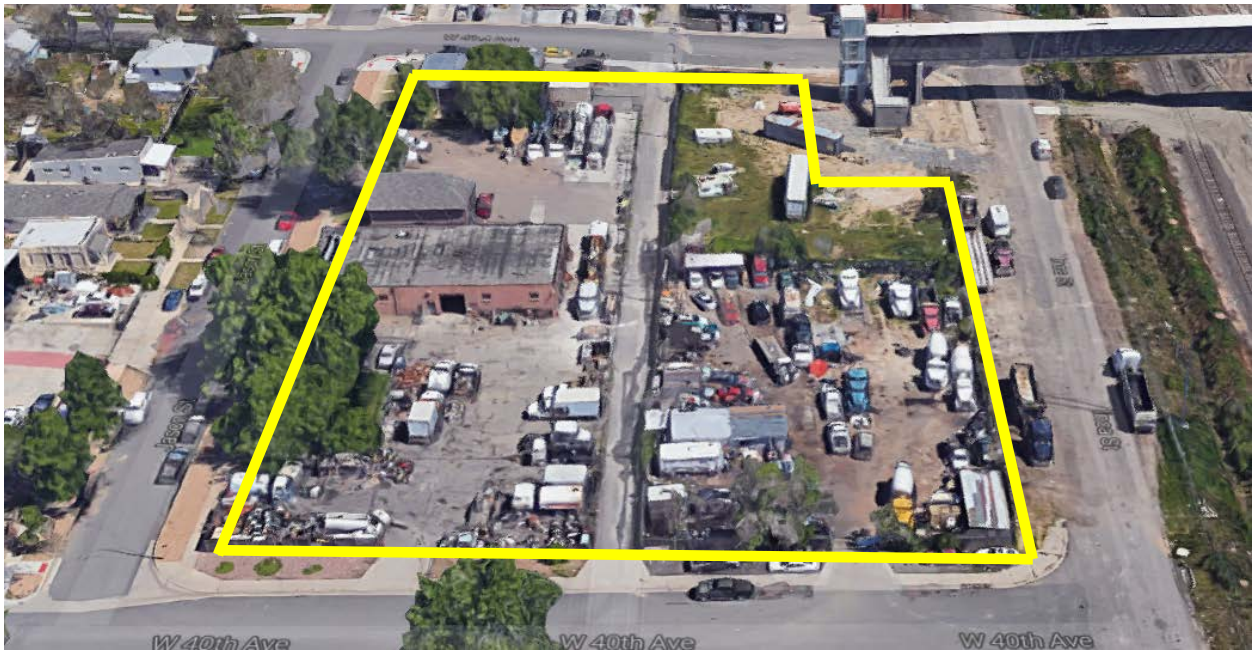
View of the site looking north, with the 41 st and Fox station area pedestrian bridge to the northeast of the site
