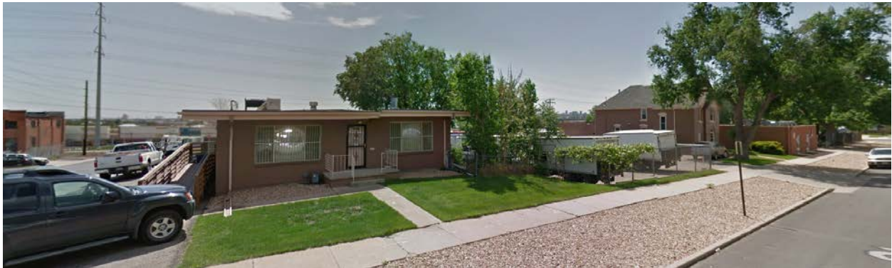
View of subject site and existing office buildings, looking east from Jason Street
