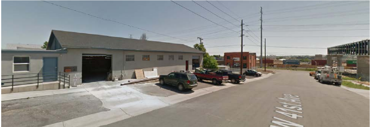
View of industrial properties north of subject site, looking east from 41 st Avenue, with the pedestrian bridge to the right
