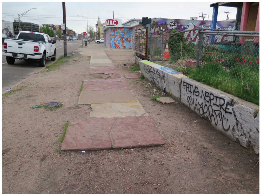
Missing and damaged flagstone sidewalk sections in front of deteriorated retaining wall
