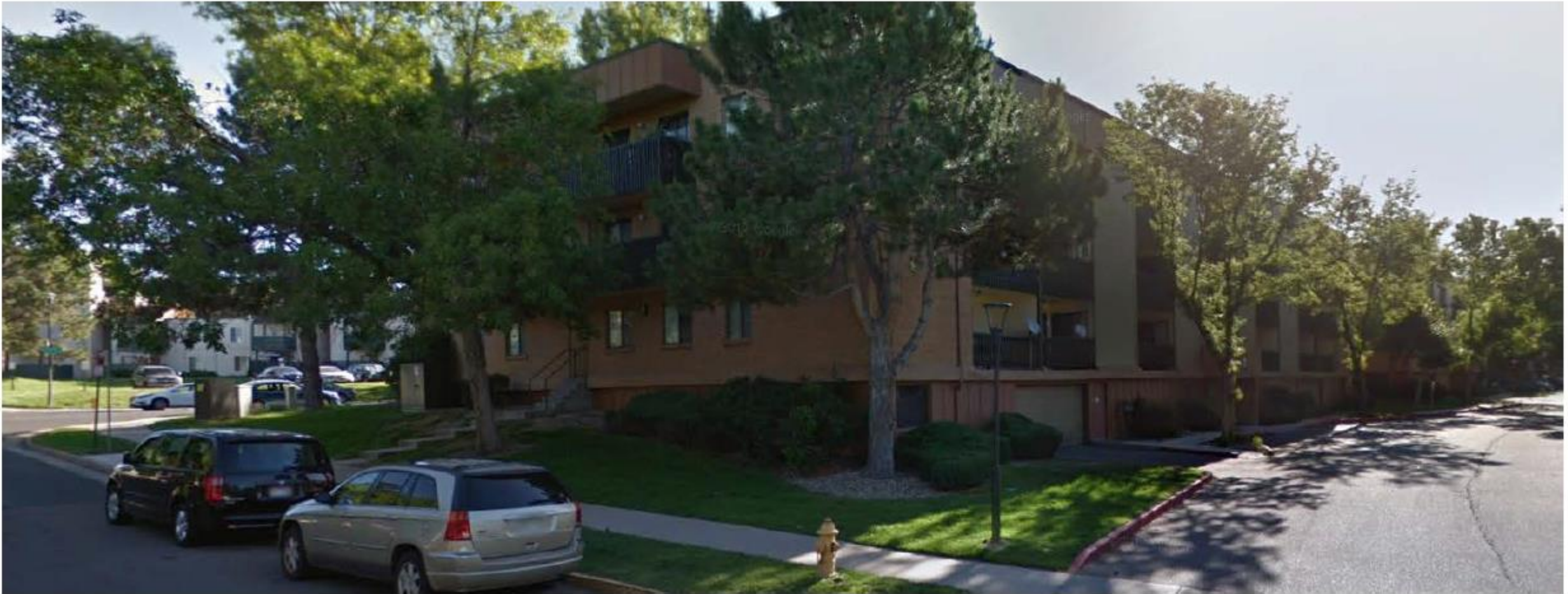
Dayton Crossing Looking East
